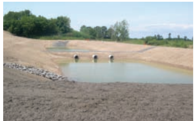
Stormwater Improvements at the Line 5 Landfill Site.
