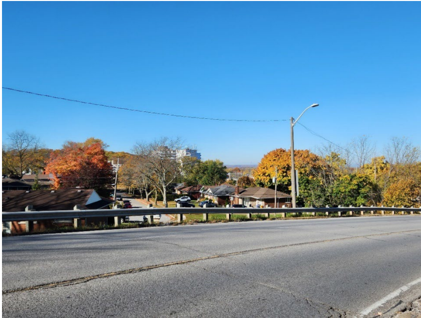
Plate 4: Protective guardrail running along the west side of Burleigh Hill Drive, looking northwest (A.S.I., 2022).
