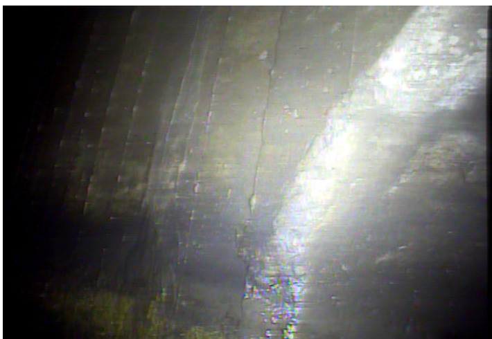
TBA - Tap, Break-in / Hammer: Active @ 0.0 m.
