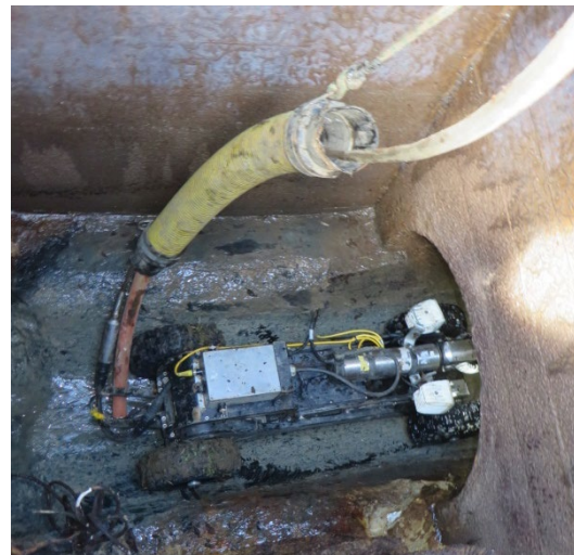
Figure 15 CCTV rover being launched at the discharge manhole of the 600 mm forcemain
