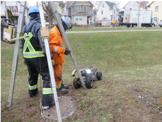
Figure 14 Setup of the CCTV rover at the discharge sewer along Palmer Avenue
