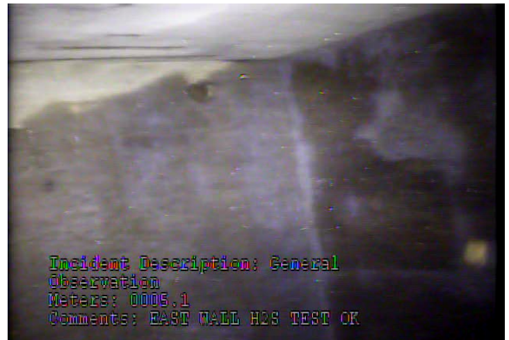
MGO - General Observation @ 5.1 m. EAST WALL H2S TEST OK
