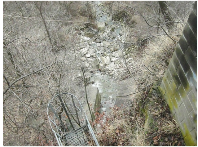
Figure 13 A view from the top of the drop shaft showing the outfall to the Niagara gorge
