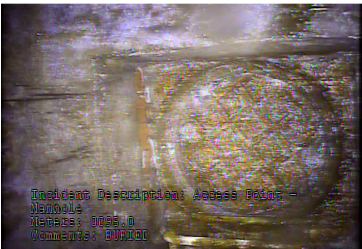
AMH - Access Point - Manhole @ 95.0 m. BURIED
