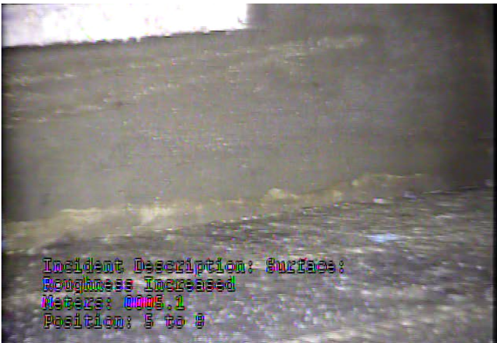
SRI - Surface: Roughness Increased @ 5.1 m.
