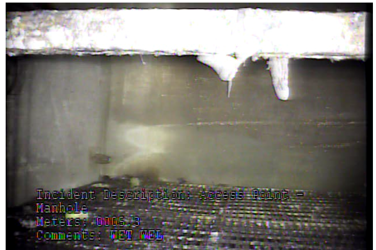
AMH - Access Point - Manhole @ 5.3 m. WET WELL
