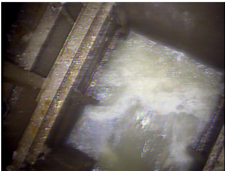
Figure 5 Observed flows at the inlet to the Bender Hill SPS wet well on April 4, 2018
