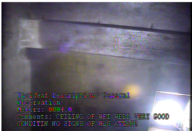
MGO - General Observation @ 4.0 m. CEILING OF WET WELL VERY GOOD CONDITIN NO SIGNS OF H2S ATTACK
