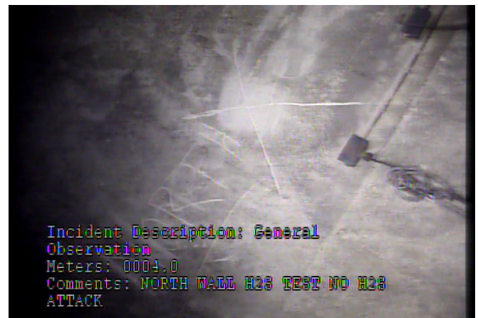
MGO - General Observation @ 4.0 m. NORTH WALL H2S TEST NO H2S ATTACK
