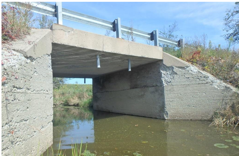
Figure 4: Creek Road Bridge
