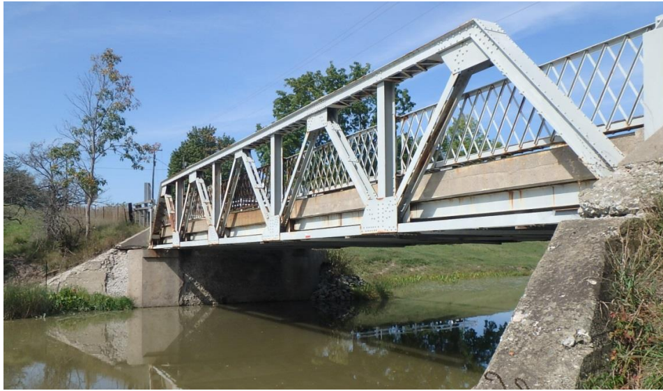
Figure 3 Oswego Creek Bridge
