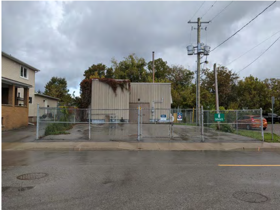
Image 1: View of Catherine Street SPS structure, exhibiting extensive disturbance, facing north
