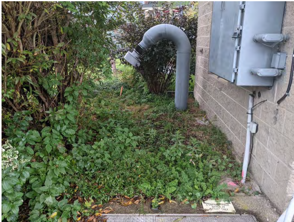
Image 12: View of landscaped garden adjacent to utilities for Lakeshore Road SPS, exhibiting archaeological potential, facing northwest
