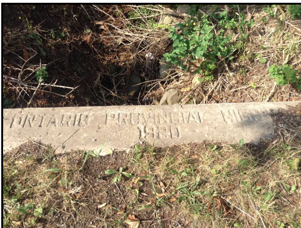
Image 12: Permanently Wet – View of culvert on King Street (Photo Taken on August 12, 2015)
