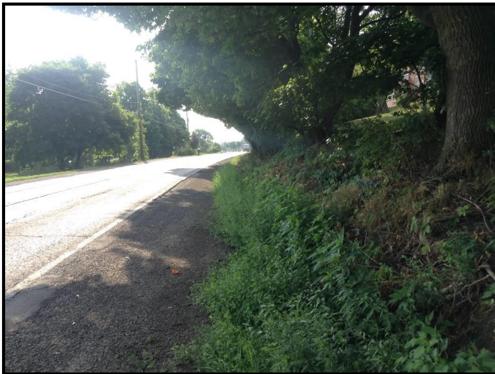
Image 11: Example of Slope on King Street (Photo Taken on August 12, 2015; Facing Southeast)
