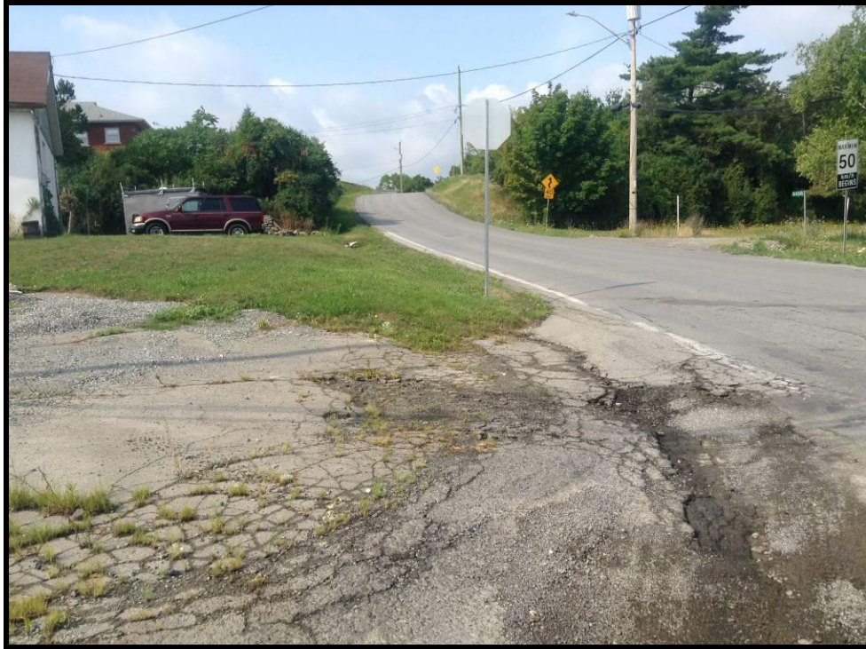
Image 9: Example of Side Street – View of Thirty Road (Photo Taken on August 12, 2015; Facing Southwest)
