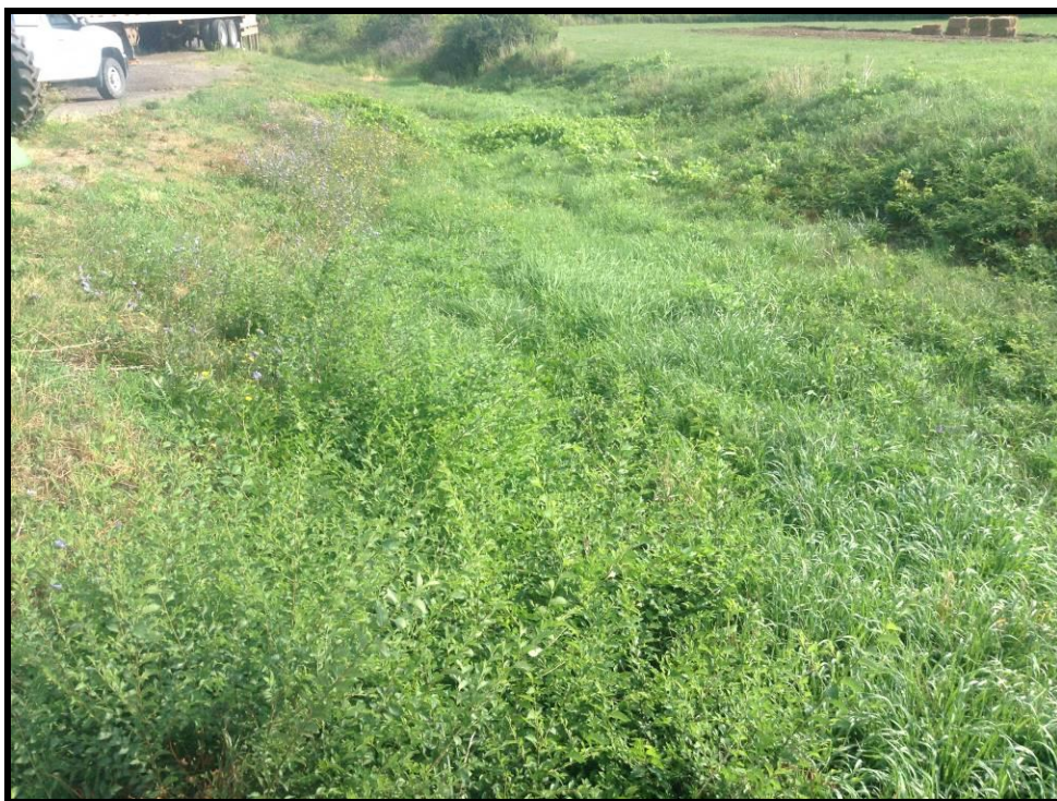
Image 14: Permanently Wet (Photo Taken on August 12, 2015; Facing North)
