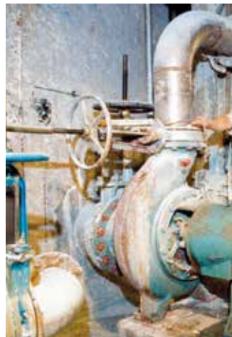
Taking suction from a large stock tank... the 3175 is the preferred pump in the Pulp & Paper Industry
