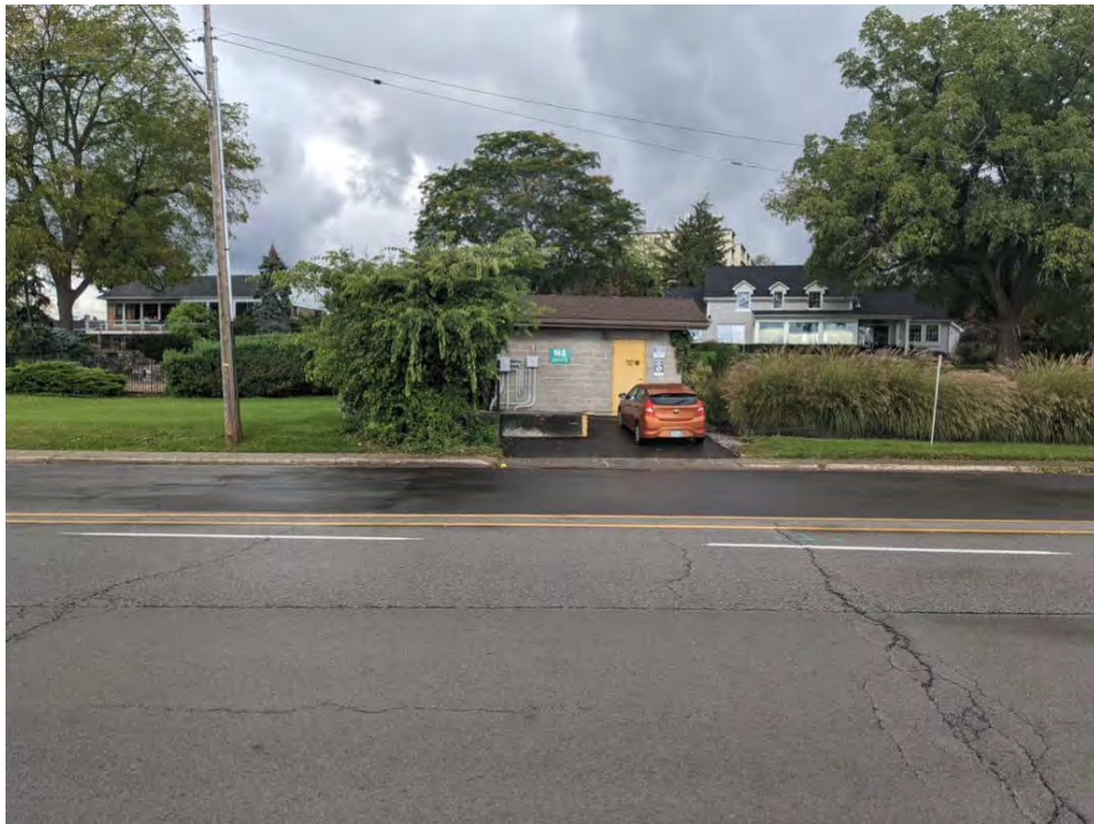
Image 8: View of Lakeshore Road SPS structure, exhibiting extensive disturbance, facing northwest
