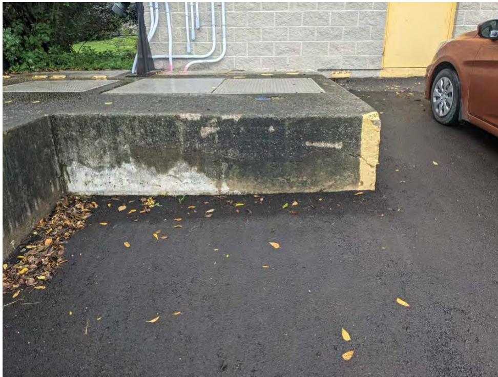
Image 11: View of short concrete platform and paved asphalt driveway for Lakeshore Road SPS, exhibiting some soil disturbance, facing northwest
