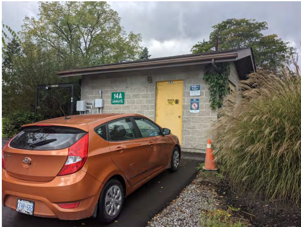
Image 9: View of Lakeshore Road SPS structure, exhibiting extensive disturbance, facing west
