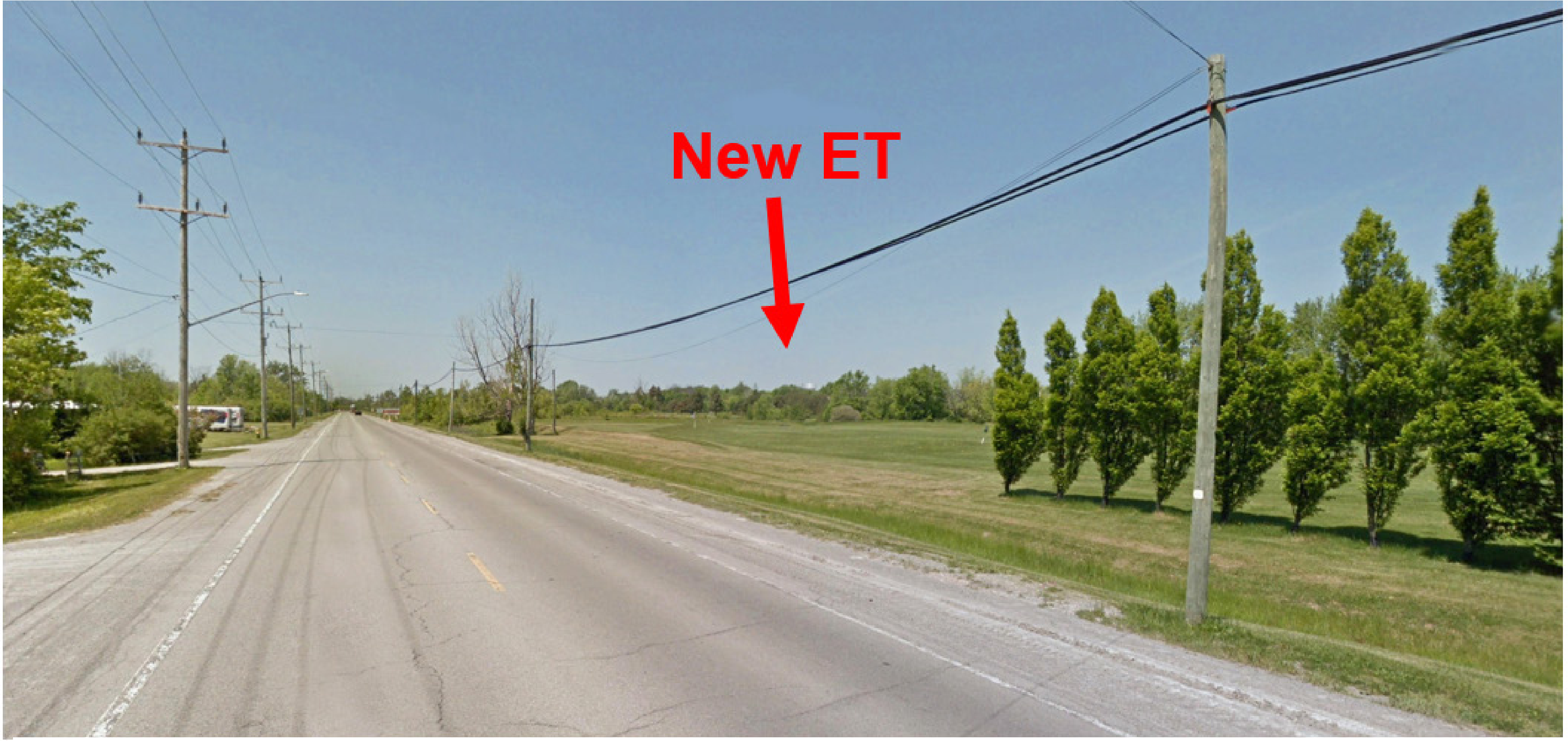
View 3 – Gilmore Road Looking North
