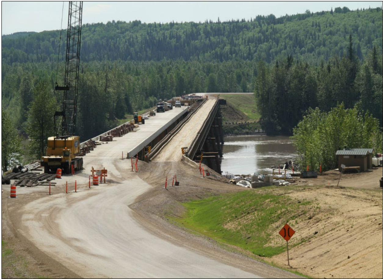
Figure 8-4: Example of Temporary Modular Bridge 22
