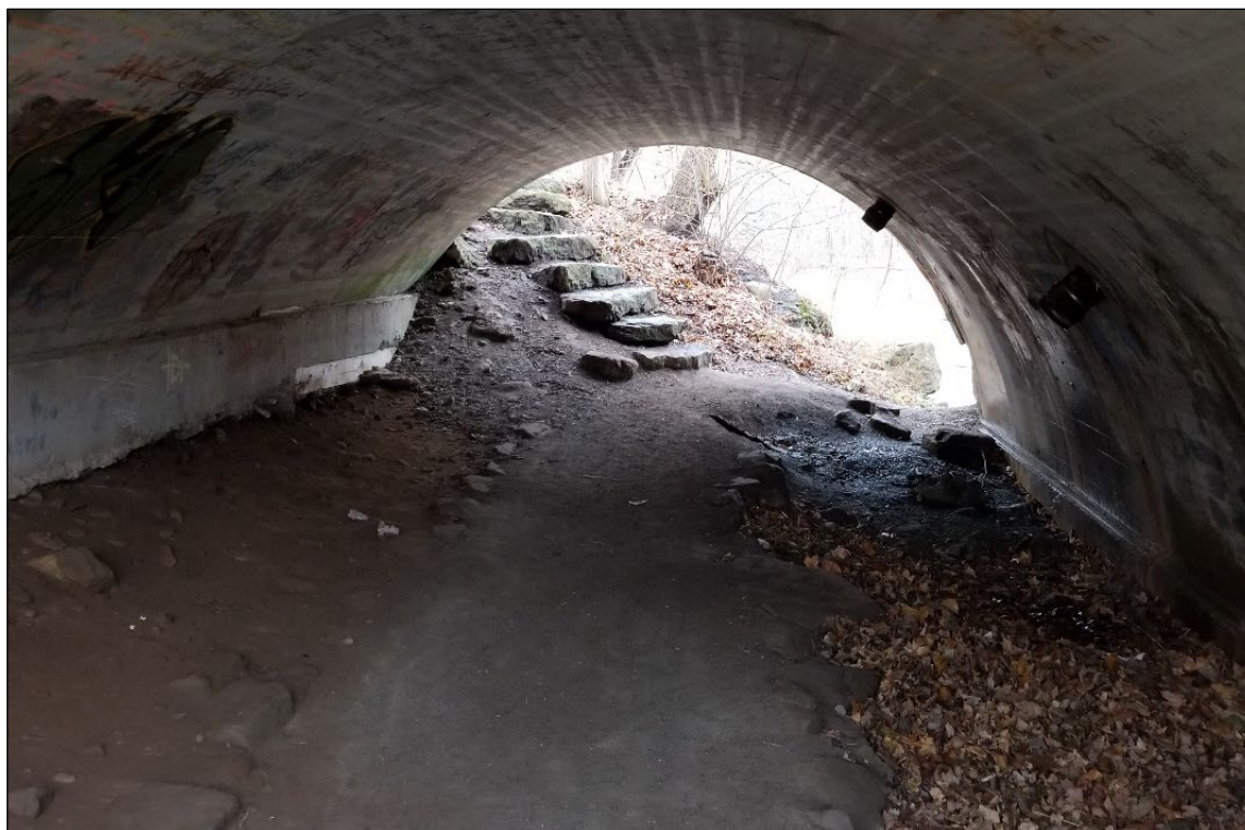
Figure 5-4: Pedestrian Path Located Under the Bridge
