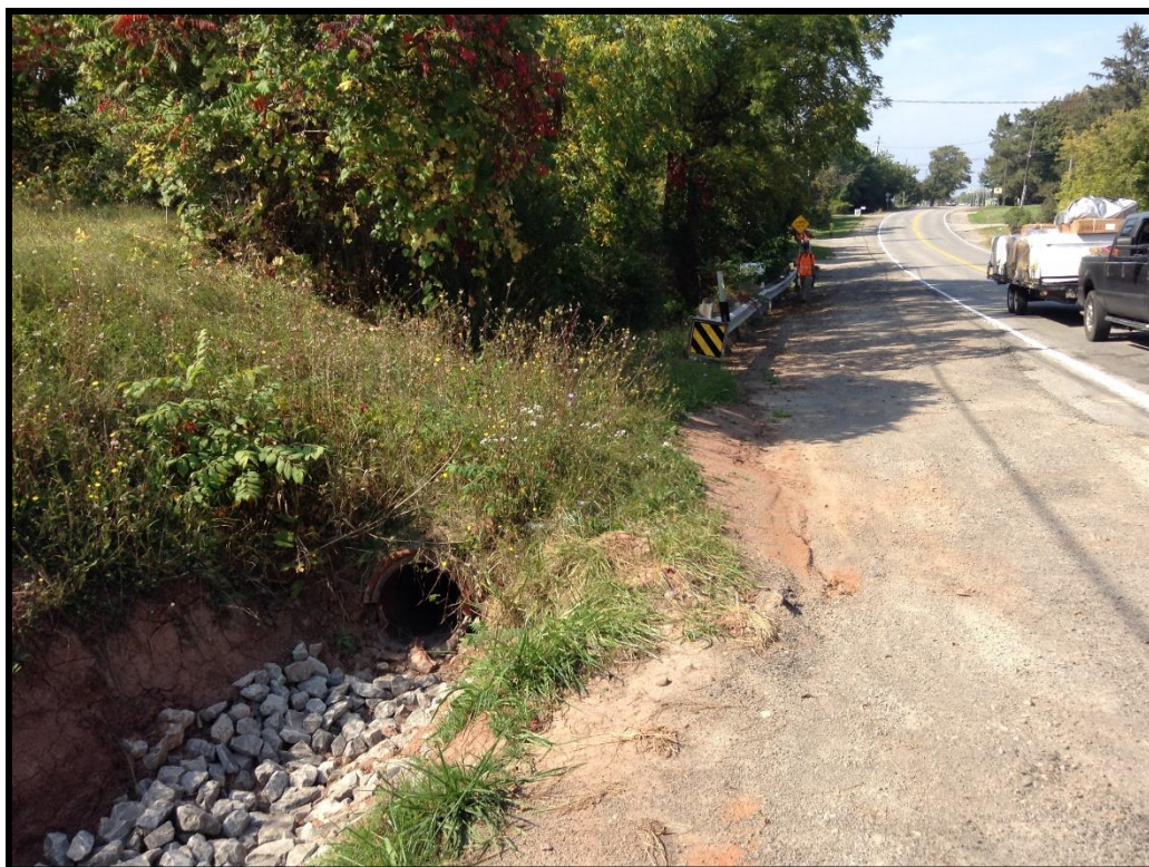
Image 7: Environs facing southeast, note gravel shoulder and culvert
