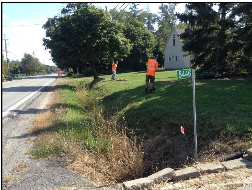
Image 11: Environs and test pit survey facing southeast, note road ditch
