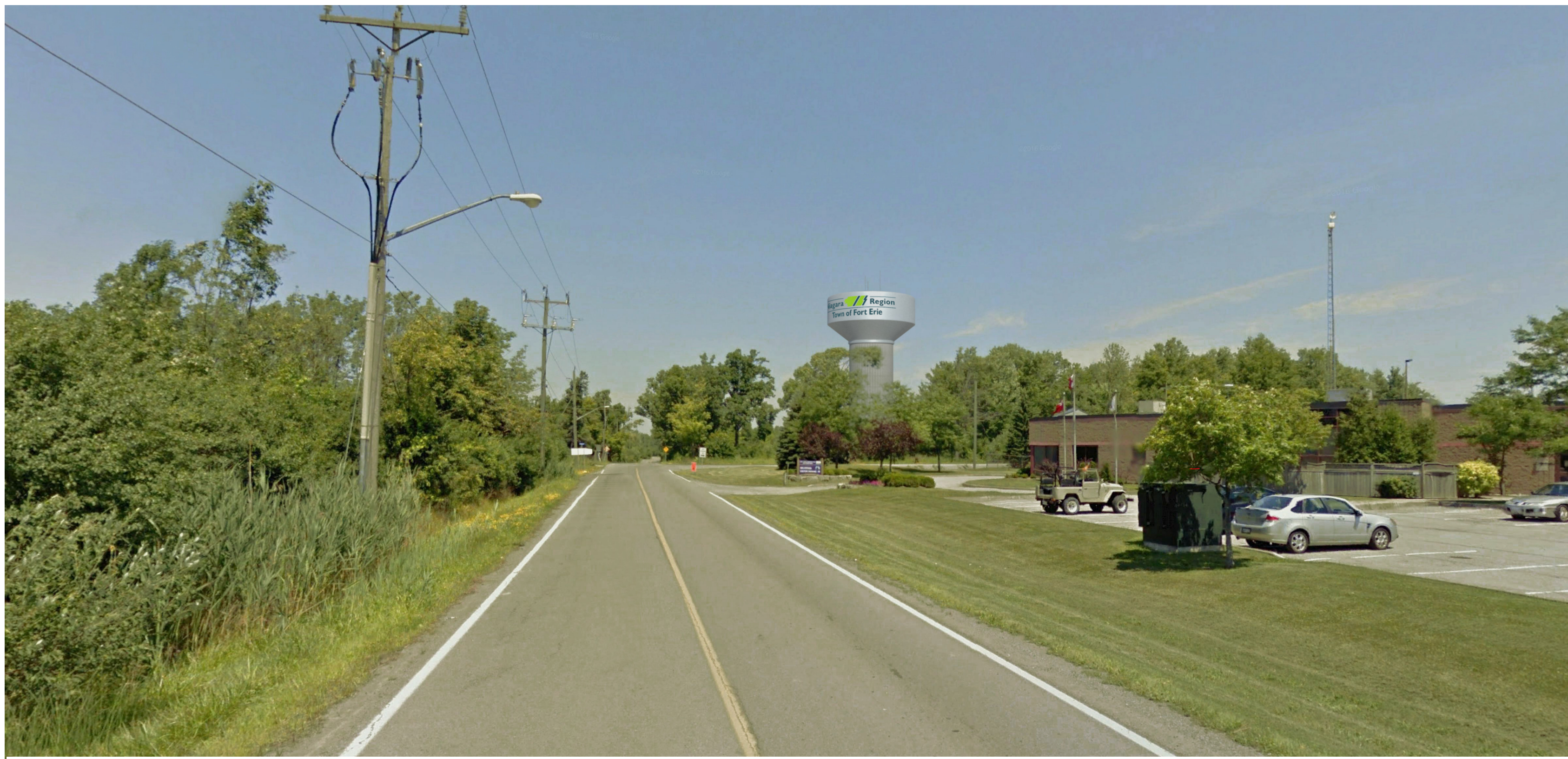
View 1 – Pettit Road Looking North Towards Bridge Street
