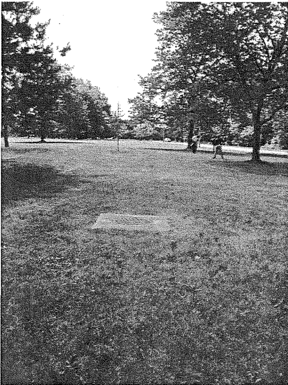
Plate 3: View southeast at disturbed area of grass covered lawn, note manhole cover.
