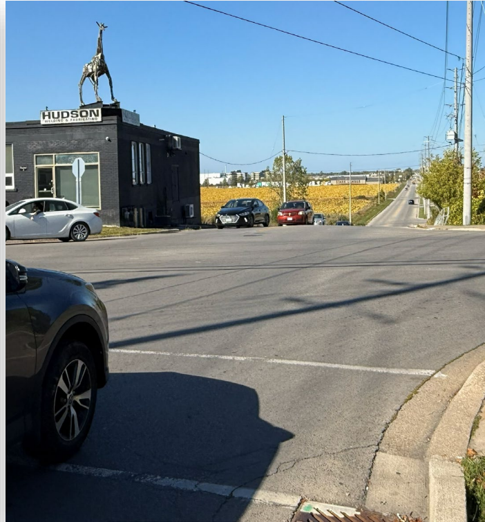
Poor visibility at the intersection going northbound.
