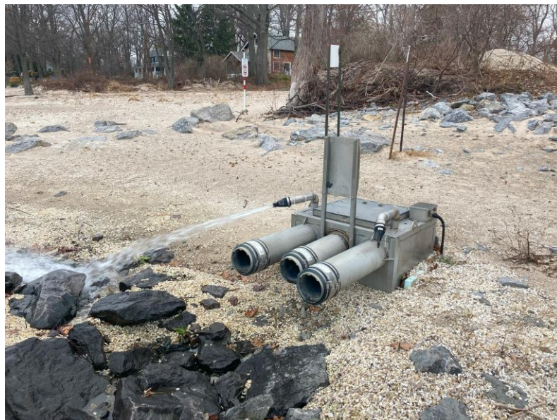
Figure 5.3: Existing Plant Drain Outfall
