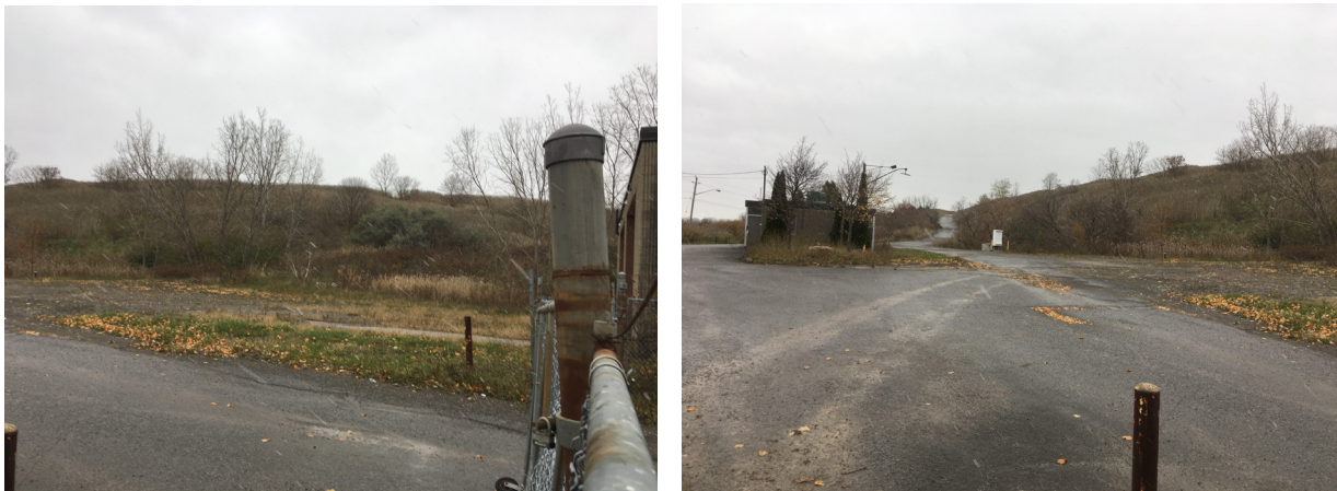
Figure 3-5. Existing Exterior Conditions
