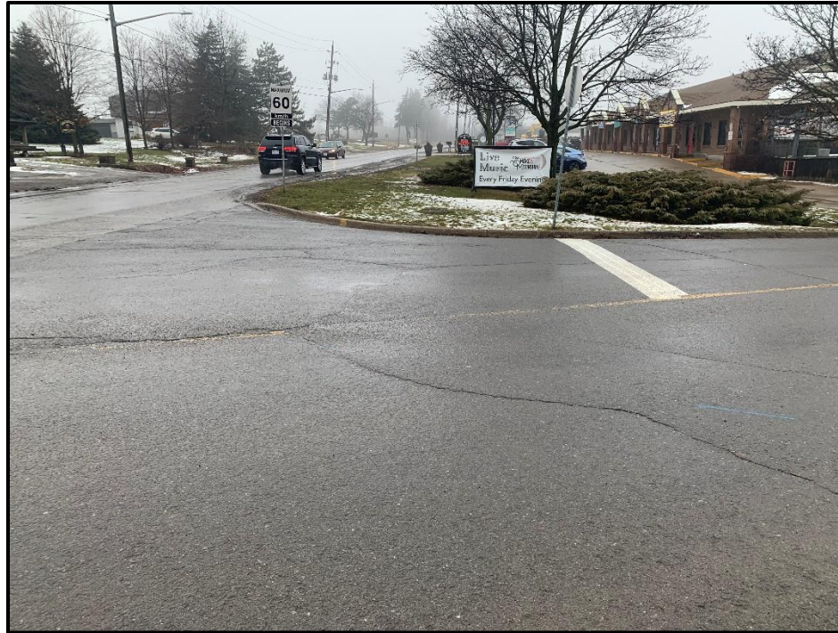
Figure 3.4 – North Approach – Stop Bar Placement
