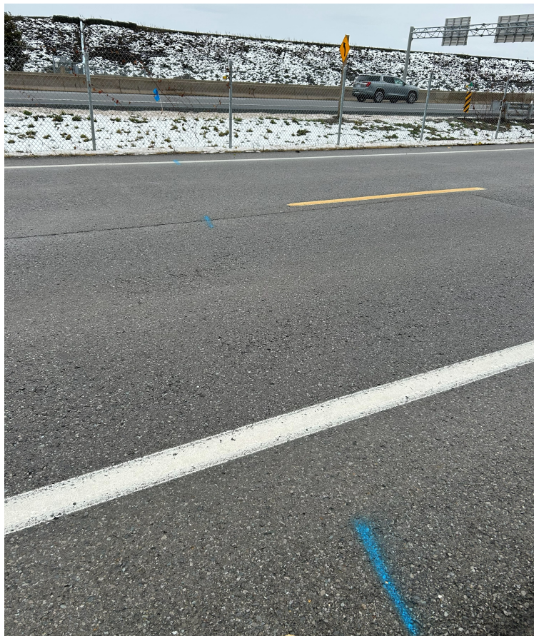
Figure 29: OPG Siphon Highway Crossing
