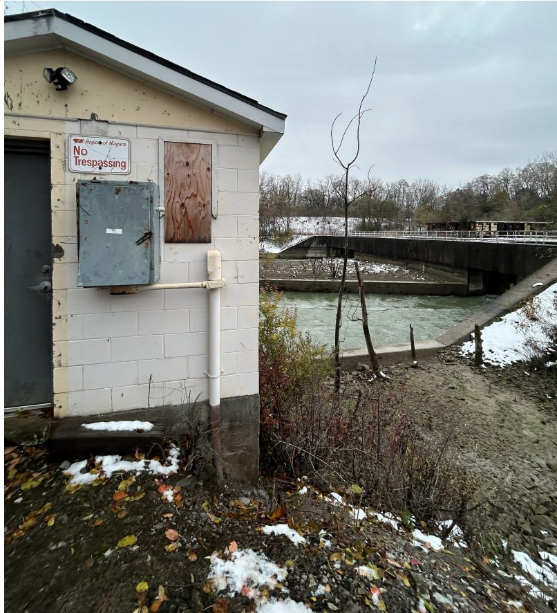
Figure 38: Existing Whirlpool Pumping Station
