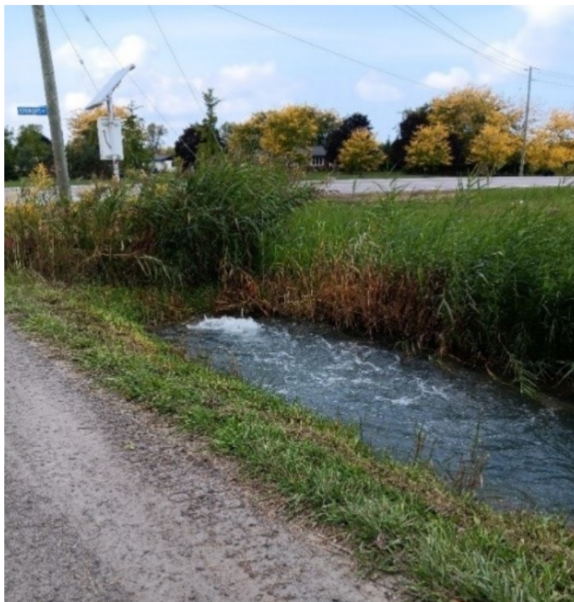
Figure 42: Irrigation Ditch with 400-millimetre Forcemain from Eastchester
