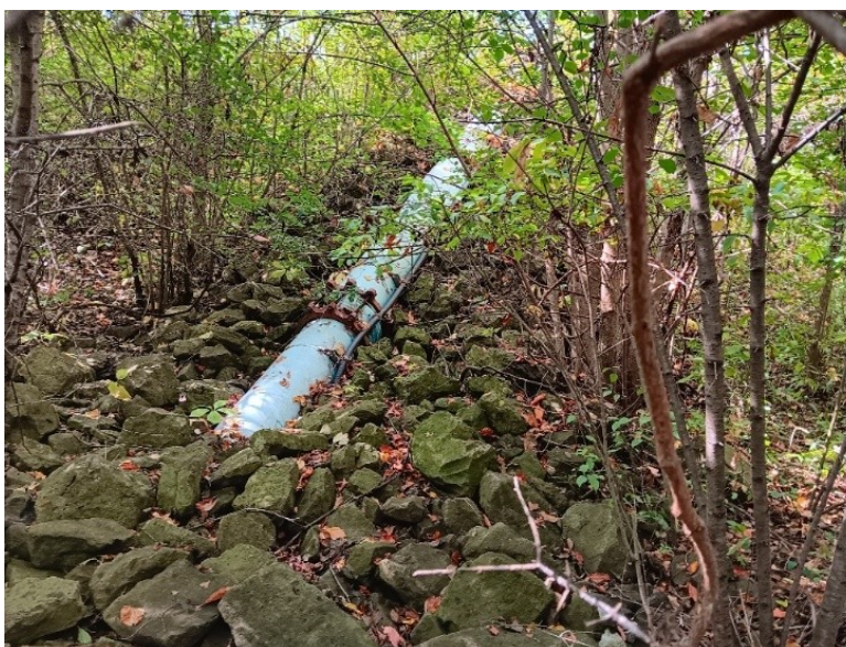
Figure 44: Existing 400-millimetre Forcemain at Eastchester Pump Station
