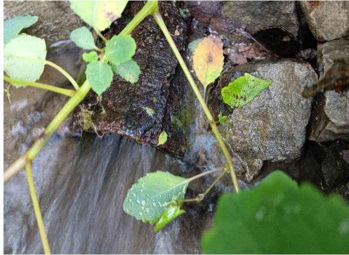
Figure 51: 150-millimetre Pipe Outlet
