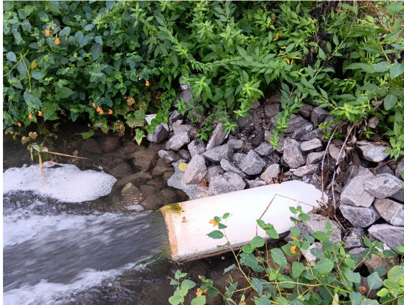
Figure 49: Discharge of Existing 200-millimetre
