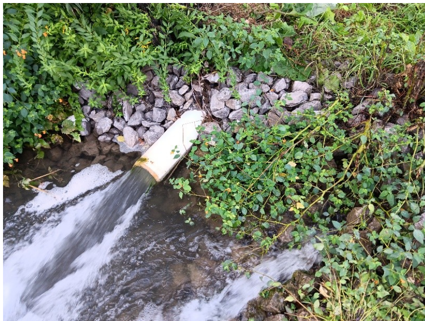
Figure 50: Water Discharges of the Decommissioned 150-millimetre Carlton Street Siphon
