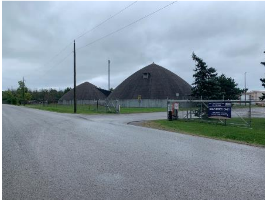
Image 29: Town of Fort Erie waste management compound immediately south of Alternative 3. Facing Southeast.
