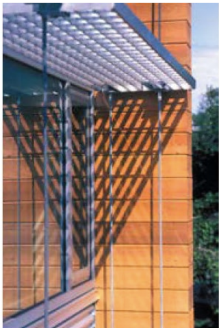
Figure: Sun louvres block high summer sun but allow low winter sunlight to enter windows.
