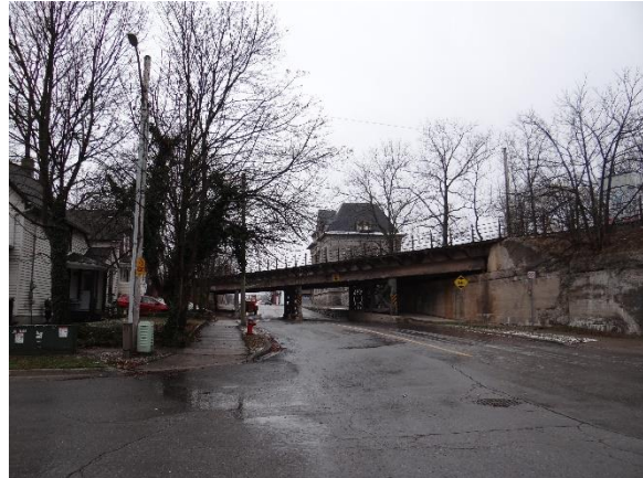
Plate 12: Park Street, looking west from Cataract Avenue (ASI 2020)
