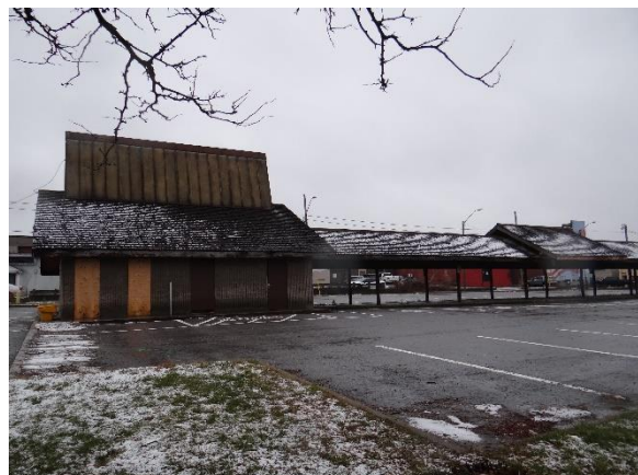
Plate 10: One of many parking lots along the south side of Park Street, looking south (ASI 2020)
