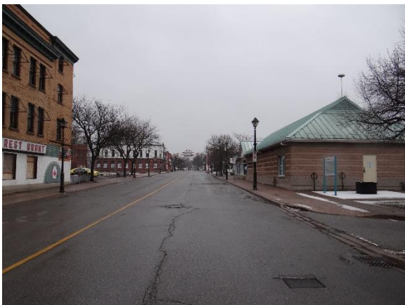
Plate 7: Erie Avenue, looking south from Bridge Street (ASI 2020)
