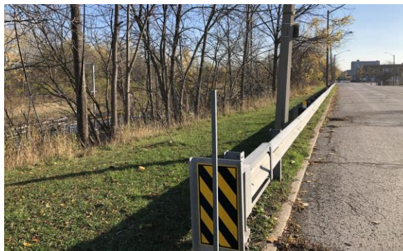
Bridge Street west of Erie north side looking eastbound
