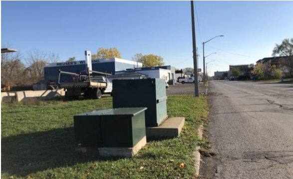
Bridge Street east of Victoria north side looking eastbound
