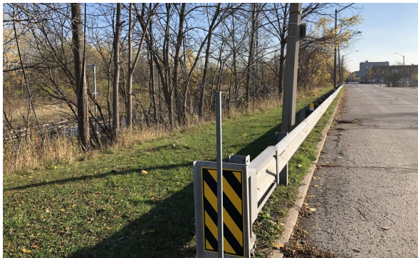
Bridge Street west of Erie north side looking eastbound
