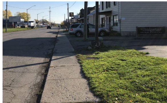
Bridge Street east of Victoria south side looking eastbound
