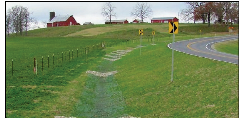
Example of Vegetative Swale with Rock Check Dams (Source: Sustainable Technologies Evaluation Program)
