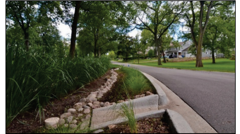
Example of Curb Cut Inlet to a Roadside Ditch LID BMP (Source: Sustainable Technologies Evaluation Program)
