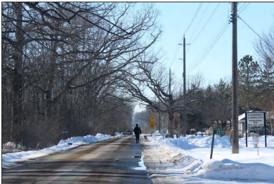
Figure 4-5: Looking westerly towards Merritt Road Segment 2
