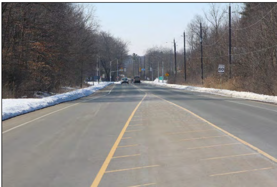
Figure 4-7: Looking westerly towards Merritt Road Segment 3
