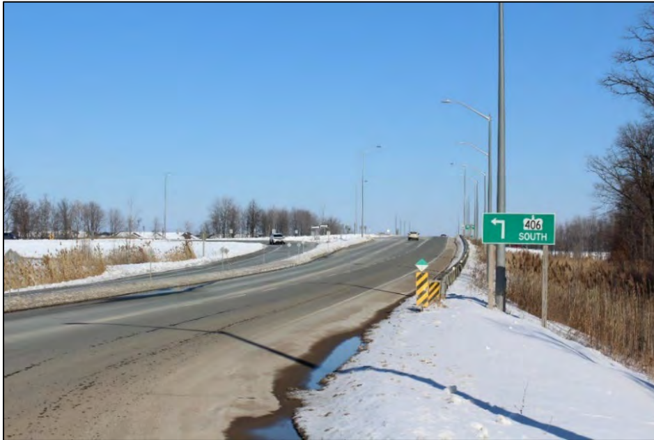
Figure 4-8: Looking easterly towards Highway 406 Interchange / Overpass Segment 3
