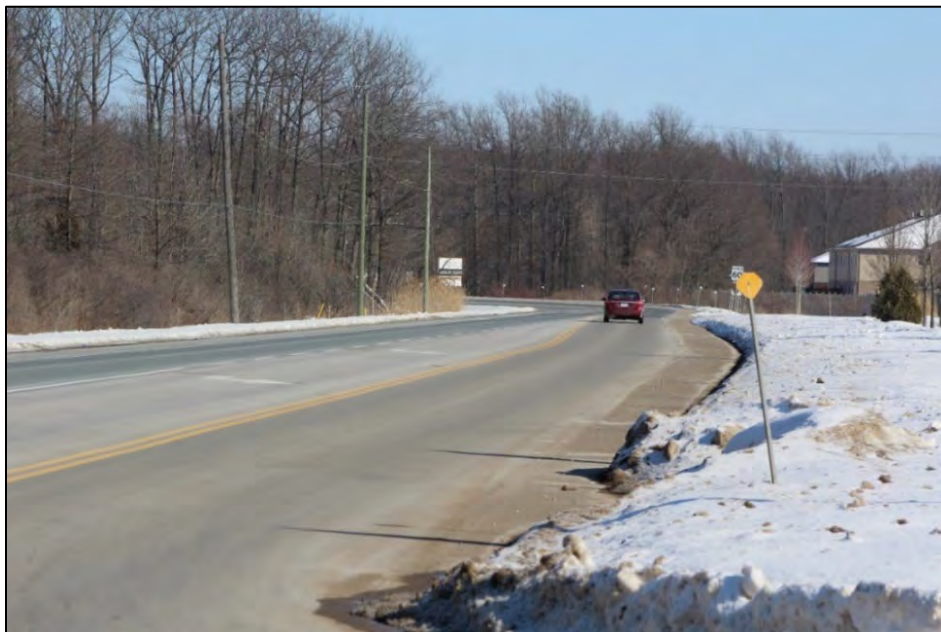
Figure 4-6: Looking easterly towards Merritt Road Segment 3
