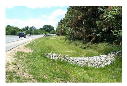
Figure 3-8 Enhanced Grass Swale (ref. Low Impact Development Stormwater Management Planning and Design Guide, Version 1.0, CVC and TRCA, 2010)
