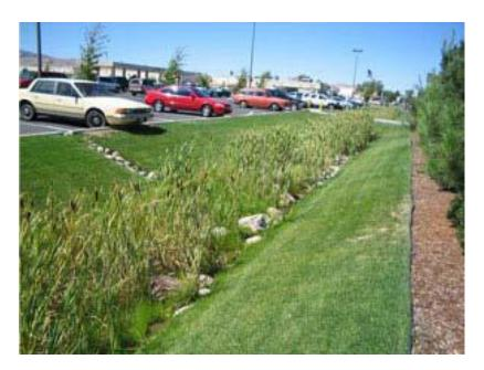
Figure 3-7 Enhanced Grass Swale (ref. Low Impact Development Stormwater Management Planning and Design Guide, Version 1.0, CVC and TRCA, 2010)
