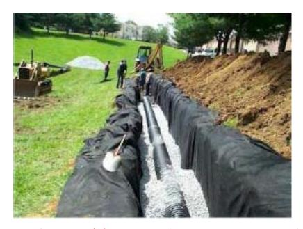
Figure 3-9 Infiltration Trench Construction (ref. Low Impact Development Stormwater Management Planning and Design Guide, Version 1.0, CVC and TRCA, 2010)
