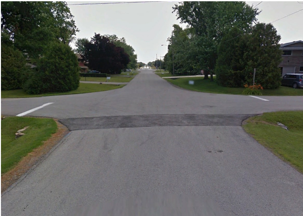
Photograph 4 – Livingston Avenue, westbound, west end of Emily Street, looking east, showing moderate patching and slight road edge cracking.
