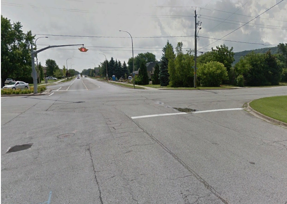
Photograph 1 – Livingston Avenue, westbound, about 10 m west of Casablanca Boulevard, looking east, showing moderate longitudinal and transverse cracking associate with moderate depression, moderate patching and slight alligator cracking.
