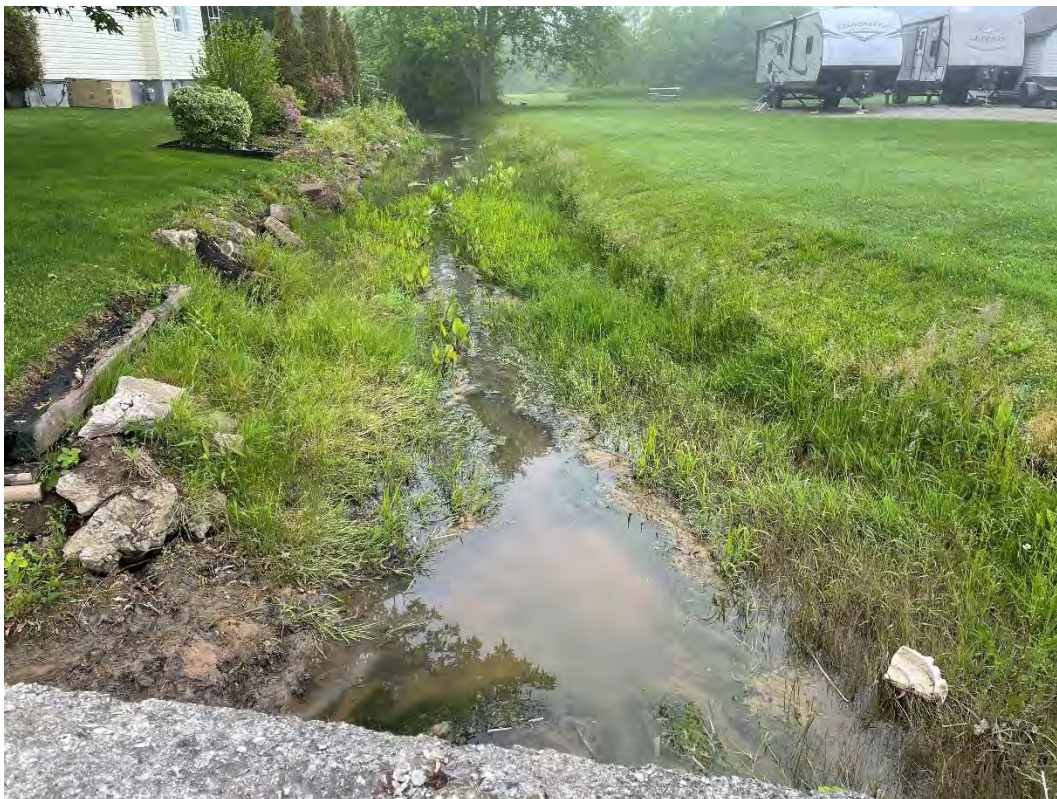
Figure 4 - East Wignell Drain at Weaver Road
