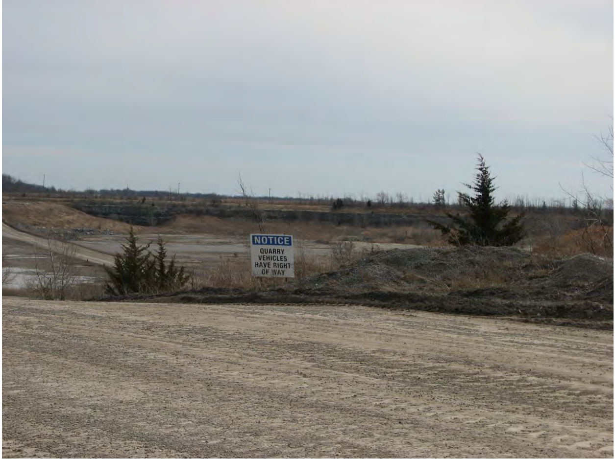
West Face of Pit 2
