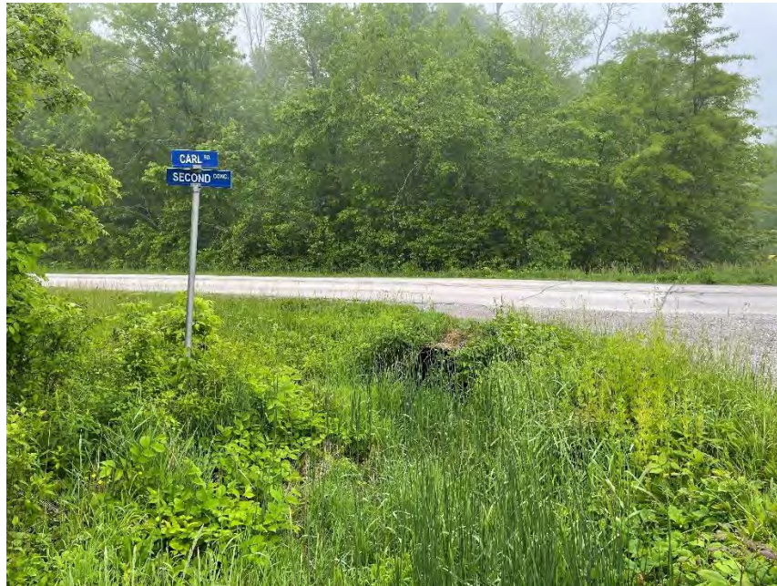
Figure 1 - Culvert under 2nd Concession Road (looking south)
