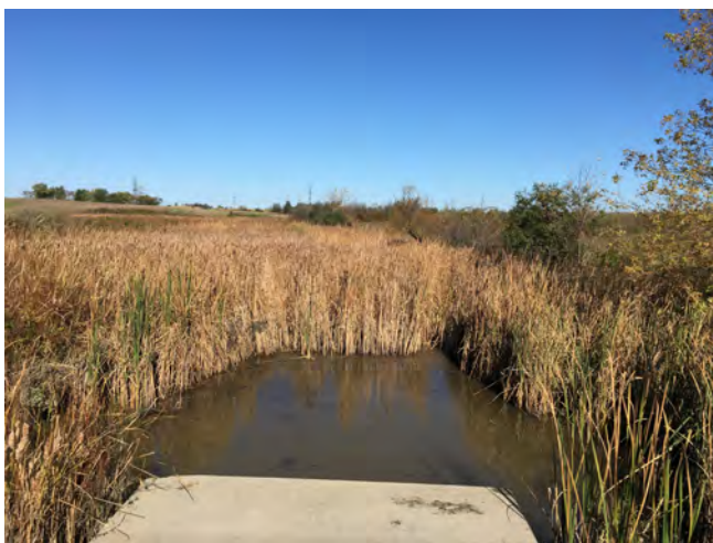
Photo 3: Looking downstream from downstream end of Uppers Lane culvert (October 2017).
