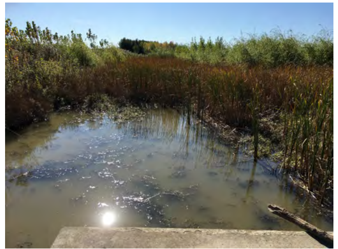
Photo 2: Looking upstream from upstream end of Uppers Lane culvert (October 2017).
