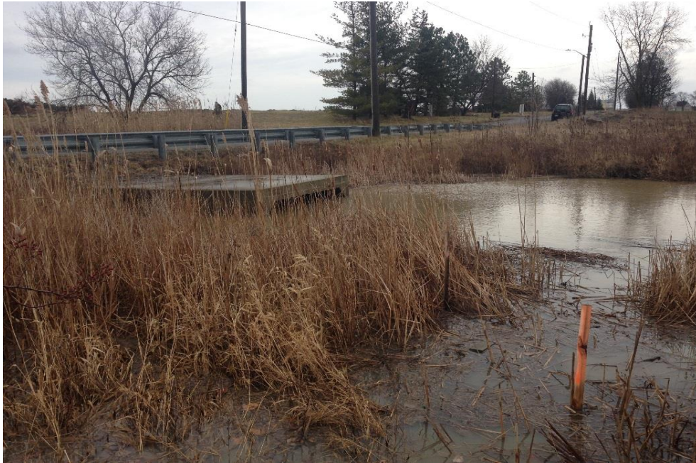
Photo taken on March 7, 2017 (looking downstream to the southeast).
