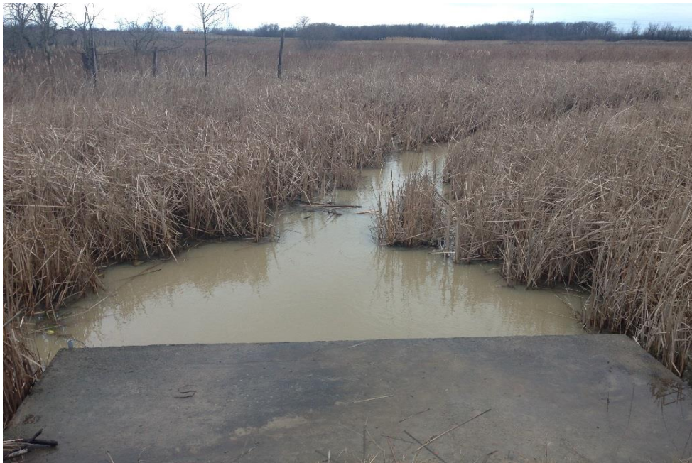
Photo taken on March 7, 2017 (looking downstream to the north).
