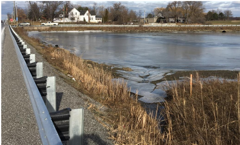
Photo taken on January 13, 2017 (looking downstream to the northeast).
