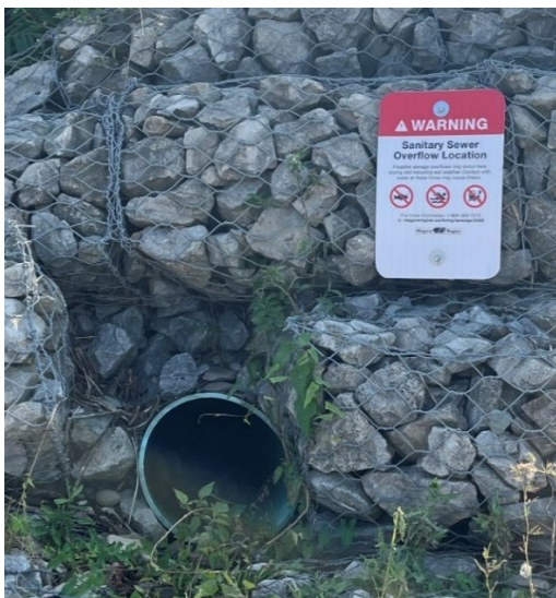
Figure NF-C- 2 - Image of Sanitary Sewer Overflow Public Signage
