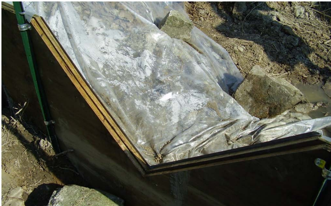
Figure 7: Detail of V-notch Facing Upstream
