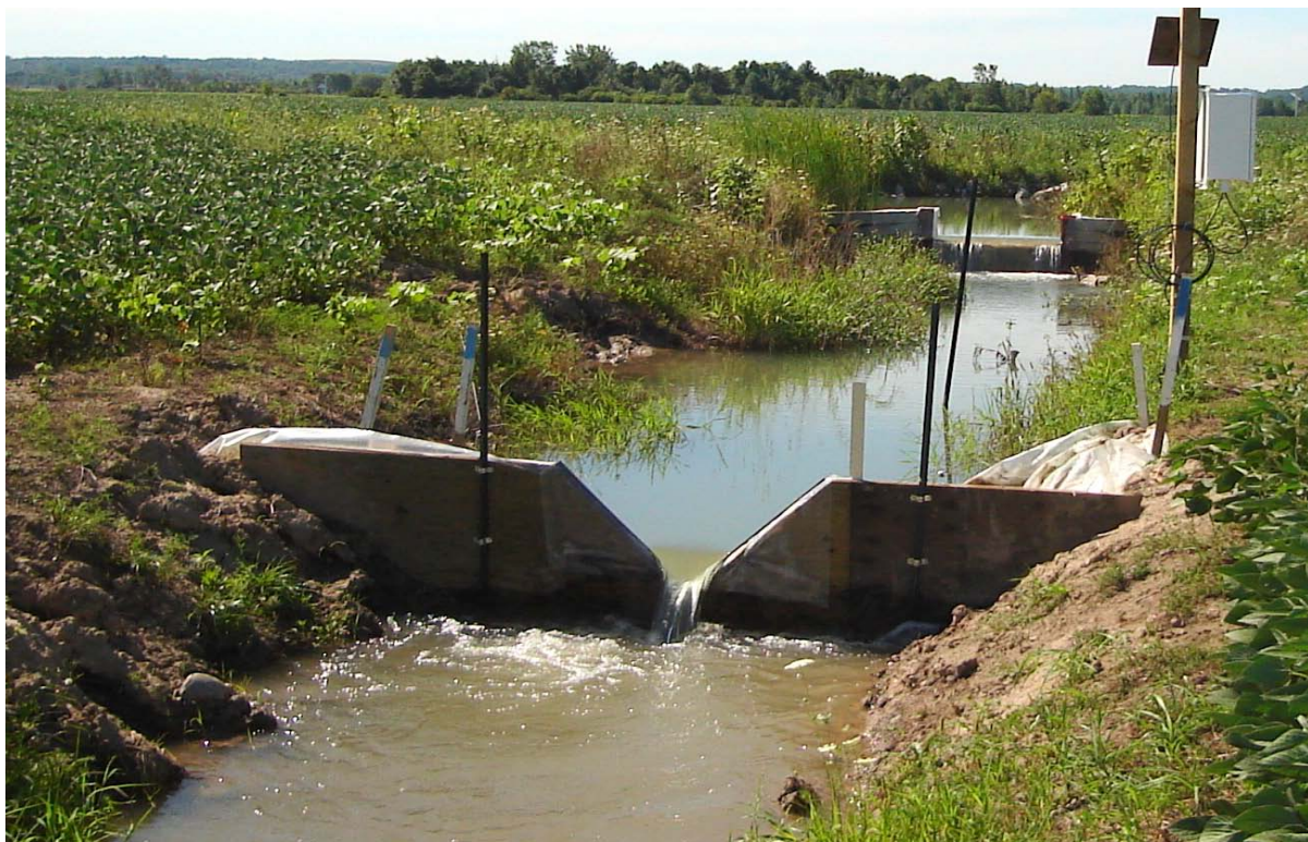
Figure 2: Top of the Lavigne Drain Looking Upstream
