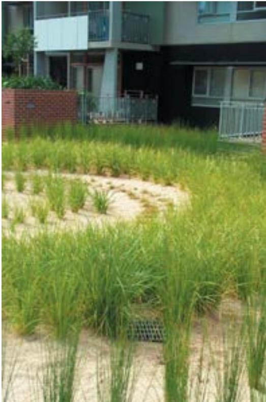
Figure: Example of bioswale incorporated within multi-unit residential development. Bioswales can be used to filter rainwater on-site.
