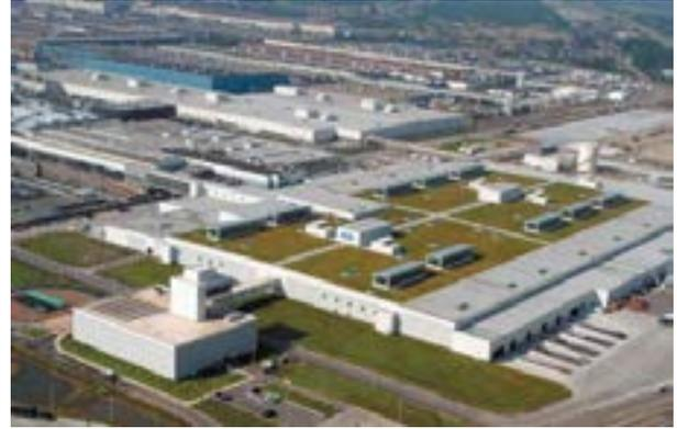
**Figure: Green roofs minimize water runoff and assist building insulation systems.**
