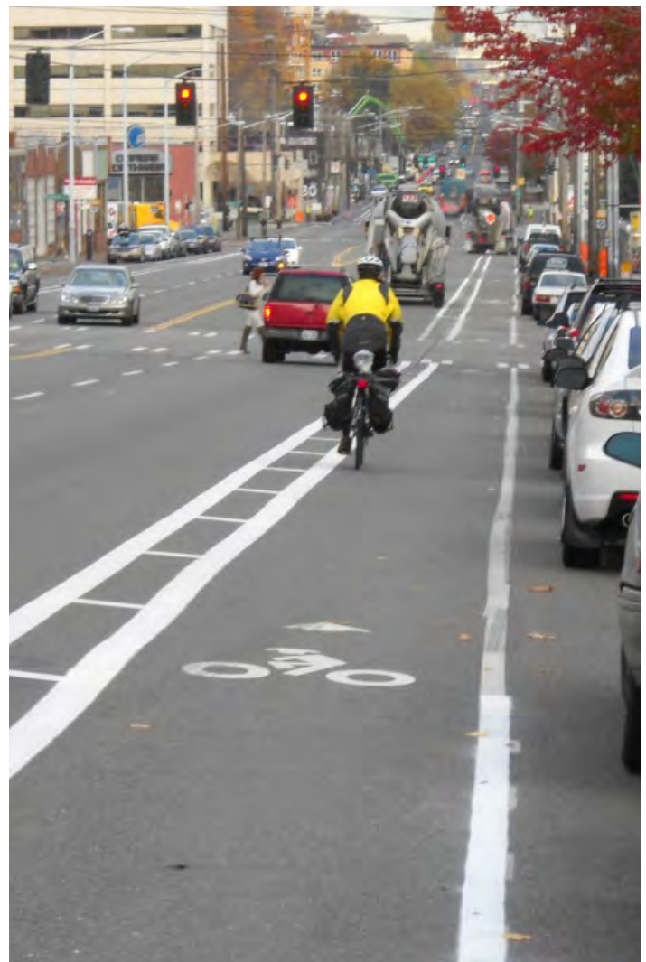
Buffered bike lanes are conventional bicycle lanes paired with a designated buffer space separating the bicycle lane from the adjacent vehicle travel lane and/or parking lane.
