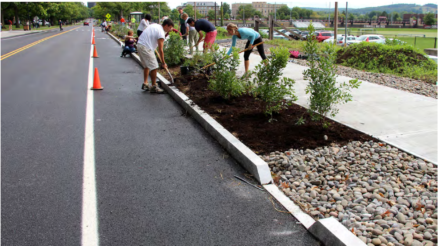
Building a bioswale adjacent to the edge zone
