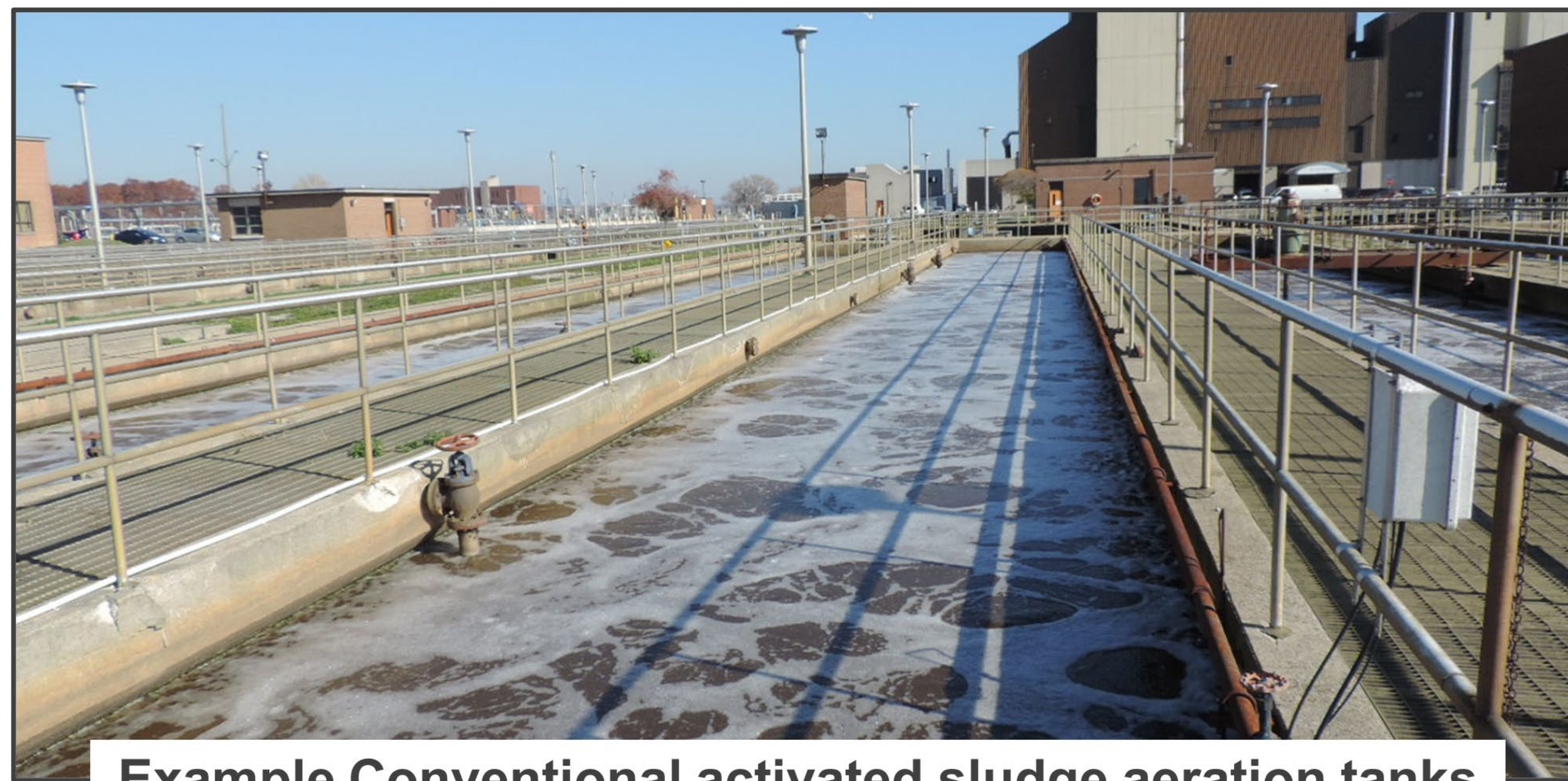
Example Conventional activated sludge aeration tanks
