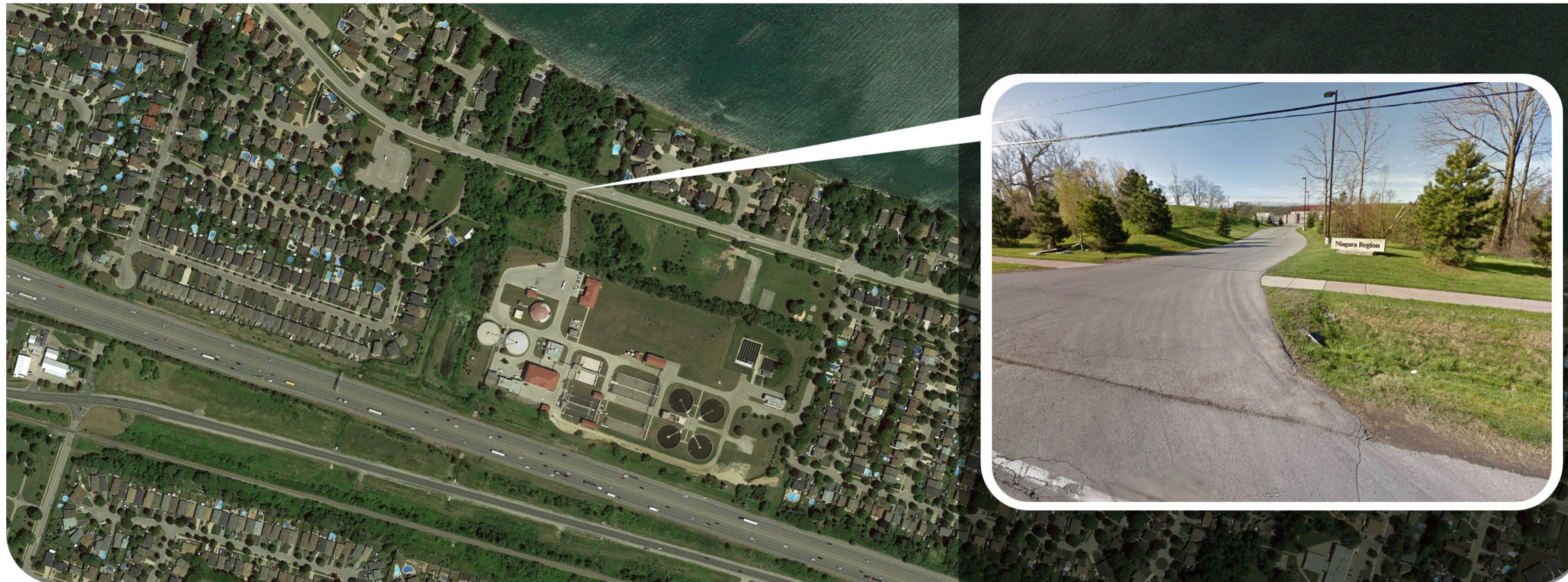
Baker Road Wastewater Treatment Plant
