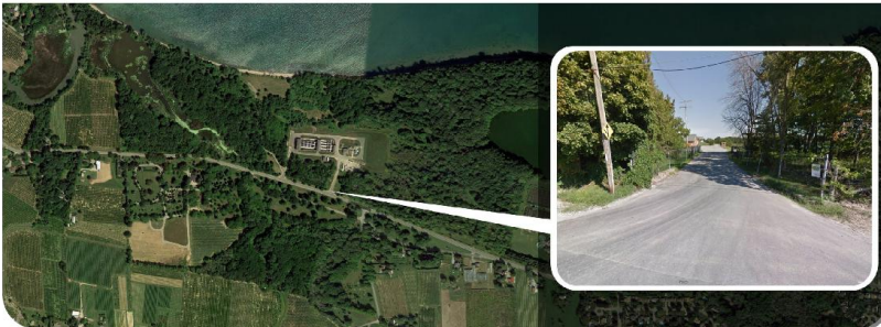
Niagara-on-the-Lake Wastewater Treatment Plant
