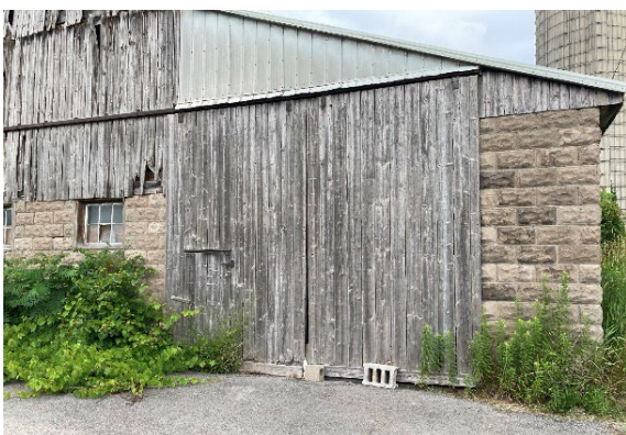
Plate 73: Sliding barn doors on the north elevation of Barn 1
