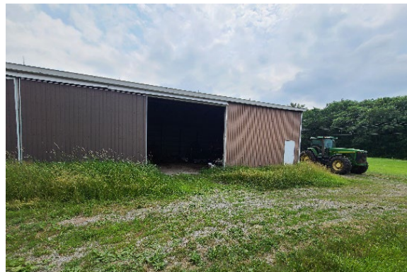
Plate 86: Outbuilding 3 with aluminium siding, west elevation
