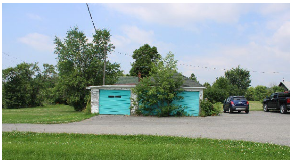
Plate 77: East elevation of Outbuilding 1 with shiplap wood siding and dual garage style doors
