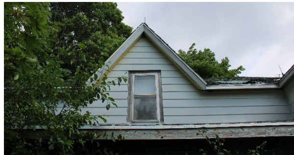
Plate 42: Sash one-over-one window found in the centre gable of the original structure on the south elevation
