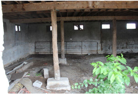
Plate 93: Interior of Barn 2
