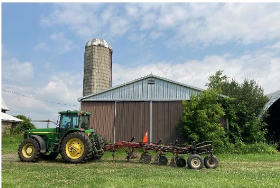
Plate 85: Outbuilding 3 with aluminium siding, south elevation
