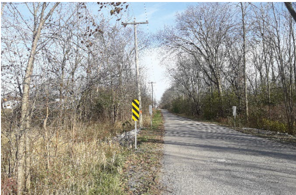
Plate 5: East view of Reixinger Road
