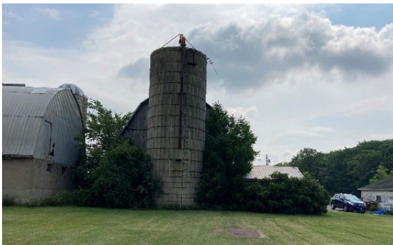
Plate 97: Precast stave Silo 1, facing east
