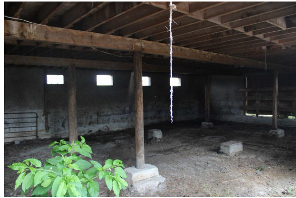
Plate 94: Interior of Barn 2
