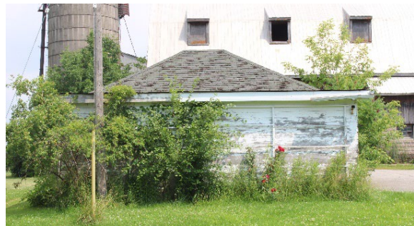
Plate 78: Southern elevation of Outbuilding 1 with shiplap wood siding
