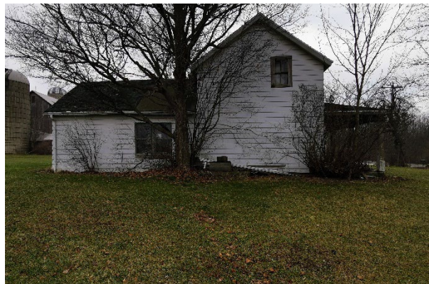
Plate 56: West elevation of 6811 Reixinger Road
