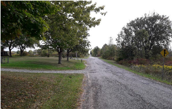
Plate 3: East view of Reixinger Road
