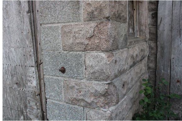
Plate 76: Concrete block and rusticated concrete block lower-level walls of Barn 1
