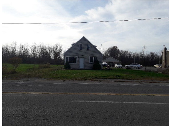
Plate 28: West view of 8760 Montrose Road (RR98)
