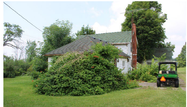
Plate 50: East elevation of 6811 Reixinger Road
