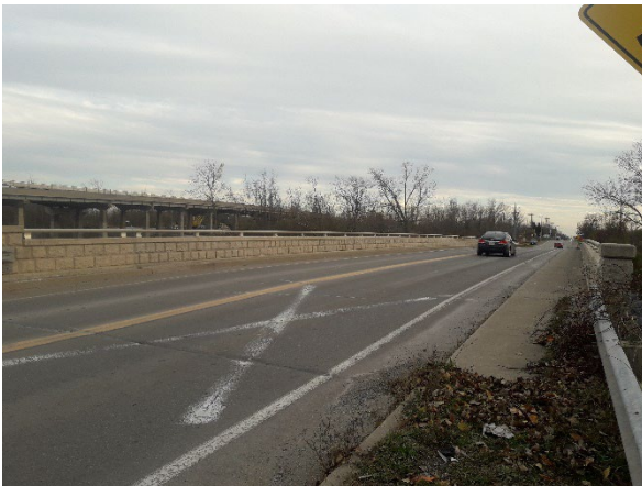
Plate 29: Northwest view of Montrose Road (RR98) Bridge
