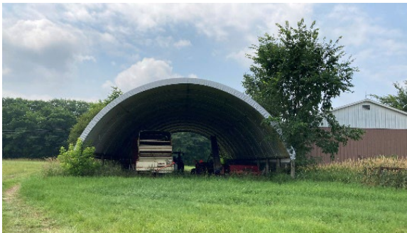
Plate 95: Open canvas style Quonset shed, facing south
