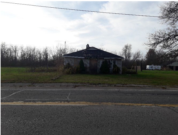
Plate 35: West view of 8762 Montrose Road (RR98)
