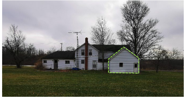
Plate 52: North elevation of 6811 Reixinger Road showing Addition C outlined in green hatching
