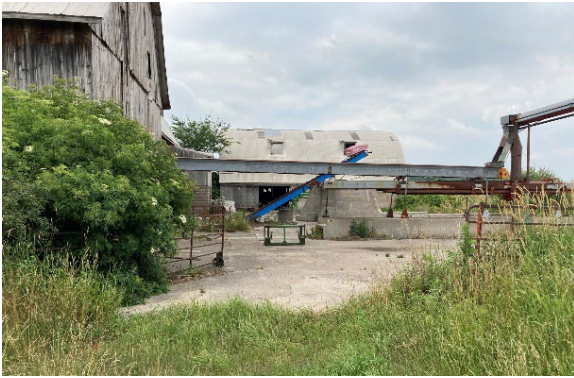
Plate 57: Metal conveyors located on the north side of Barn 1
