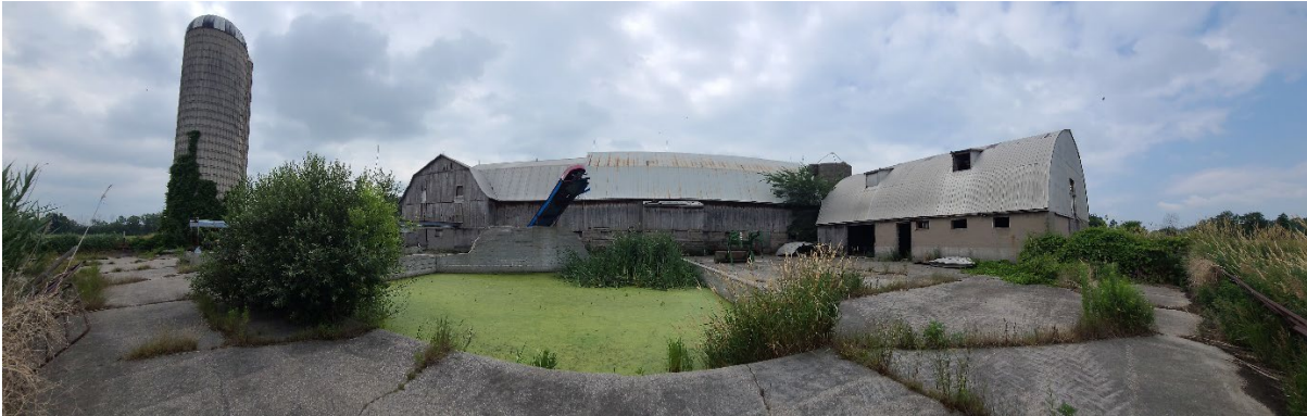
Plate 66: North elevation of Barn 1 at 6811 Reixinger Road. Silo 2 is located on the left (east), the slurry pit is located in the centre, and Barn 2 is located on the right (west)
