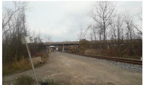
Plate 20: Northeast view of CN Railway from Montrose Road (RR98)
