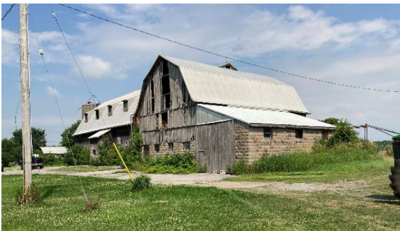
Plate 67: South and east elevations of Barn 1 at 6811 Reixinger Road
