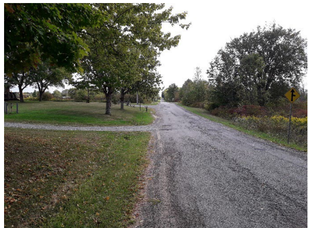
Plate 6: East view of Reixinger Road
