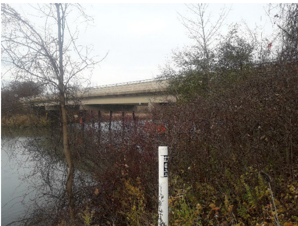
Plate 31: Northeast view of Montrose Road Bridge
