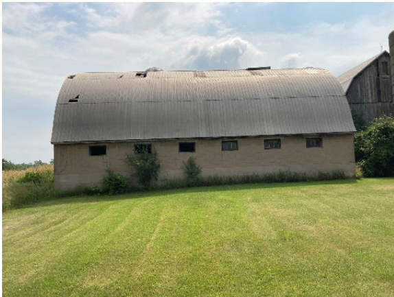
Plate 89: Barn 2 with concrete foundations/blocks and gothic arch aluminium roof, west elevation
