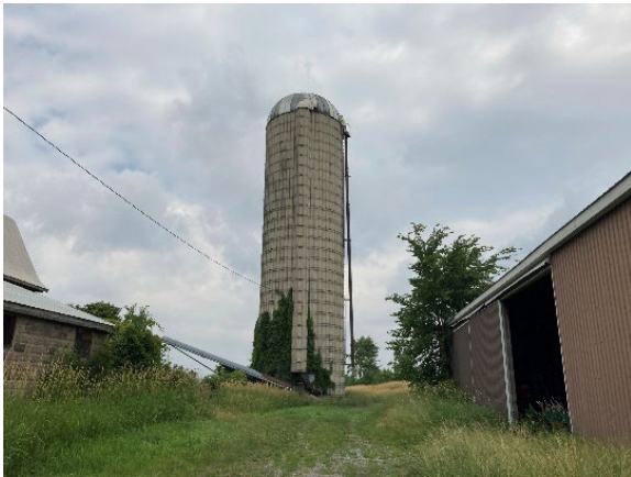
Plate 99: Precast stave Silo 2, facing north
