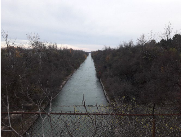
Plate 21: View of the Power Canal associated with Sir Adam Beck from McLeod Road Bridge
