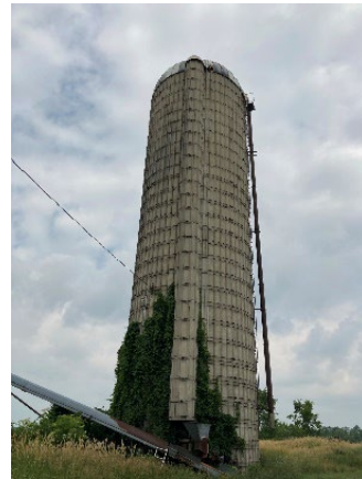
Plate 100: Precast stave Silo 2, facing north-northwest
