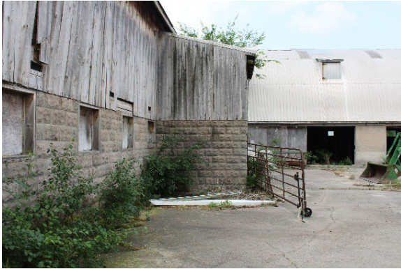
Plate 75: View of rusticated concrete block foundation of Barn 1
