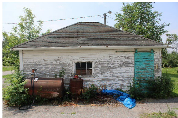
Plate 80: Northern elevation of Outbuilding 1 with shiplap wood siding sliding barn door
