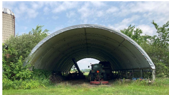
Plate 96: Open canvas style Quonset shed, facing north
