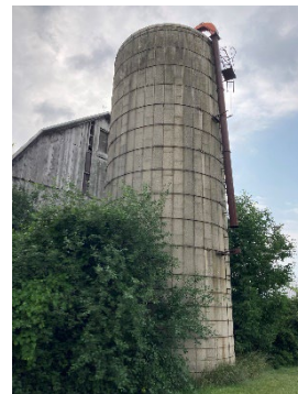
Plate 98: Precast stave Silo 1, facing southeast
