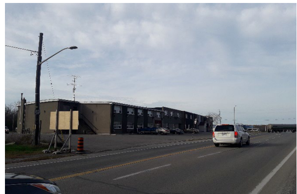
Plate 8: Northwest view of Montrose Road (RR 98) looking towards 8675 Montrose Road
