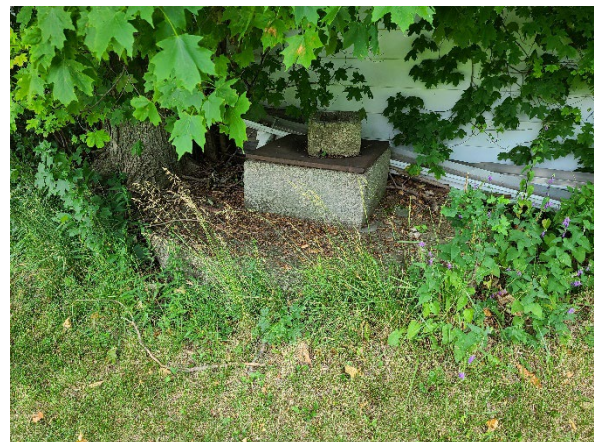
Plate 11: Concrete located along the
