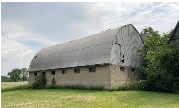
Plate 91: Barn 2 with concrete foundations/blocks and aluminium roofing, south and west elevations
