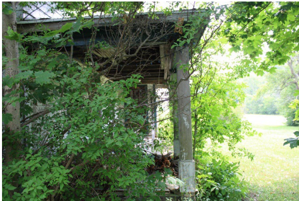
Plate 47: Covered veranda supported by wood pillars, facing southeast
