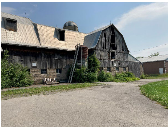
Plate 69: Barn 1 with vertical board siding, rusticated concrete block foundations, facing northeast
