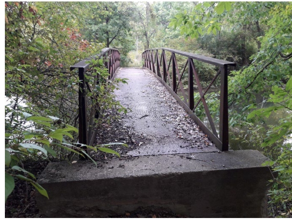
Plate 14: Metal Howe Truss bridge crossing the Welland River
