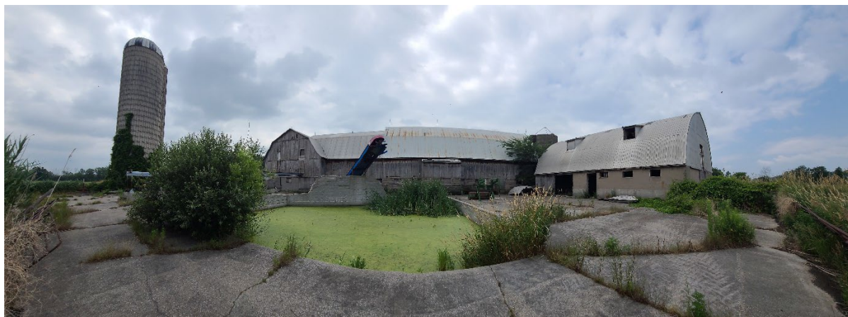
Plate 21: View of rear concrete pad and farm equipment remnants north of Barn 1 (centre) and Barn 2 (right)
