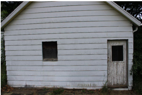
Plate 55: North elevation of Addition C
