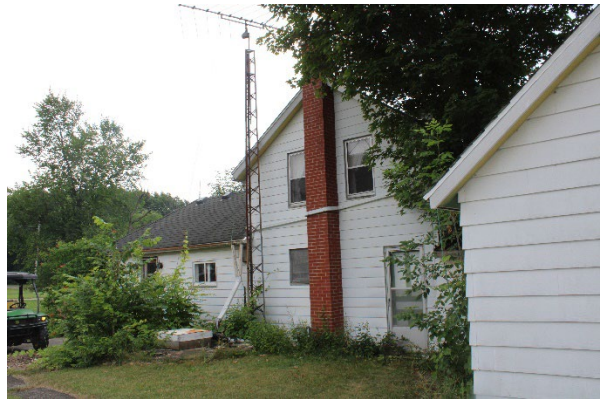
Plate 54: Exterior chimney located on the north elevation of Addition A
