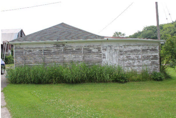
Plate 79: Western elevation of Outbuilding 1 with shiplap wood siding and wooden side door
