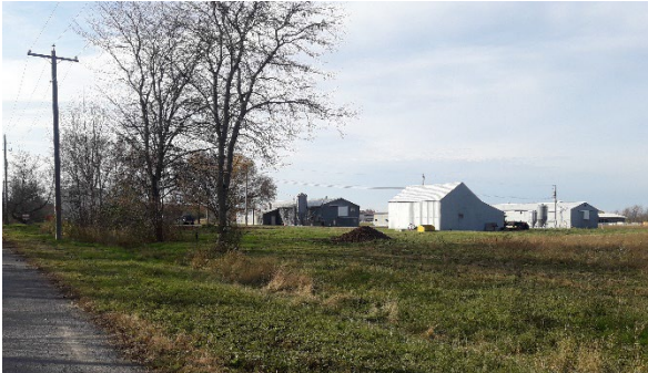
Plate 23: North view of 7473 Reixinger Road farm complex
