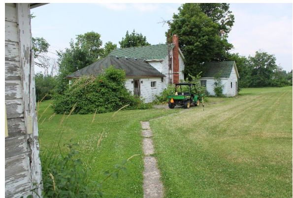
Plate 9: Concrete pathway to the main residence from the driveway facing southwest
