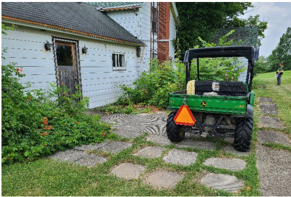
Plate 53: Concrete pad located on east side of the north elevation
