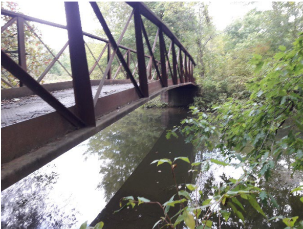
Plate 15: Metal Howe Truss bridge crossing the Welland River
