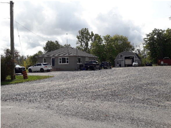
Plate 19: Southeast view Nexterra Substructures Inc. located at 7226 Reixinger Road
