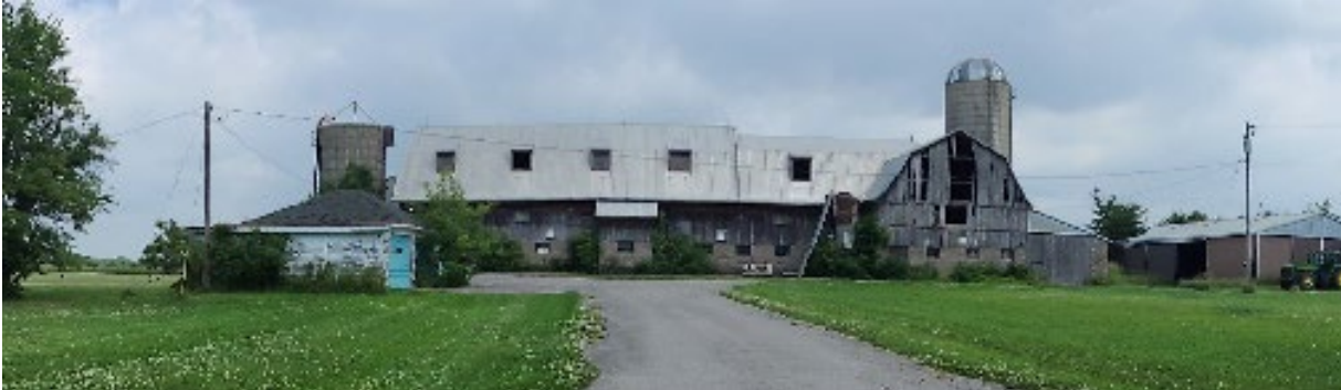
Plate 65: Front façade (south elevation) of Barn 1 at 6811 Reixinger Road
