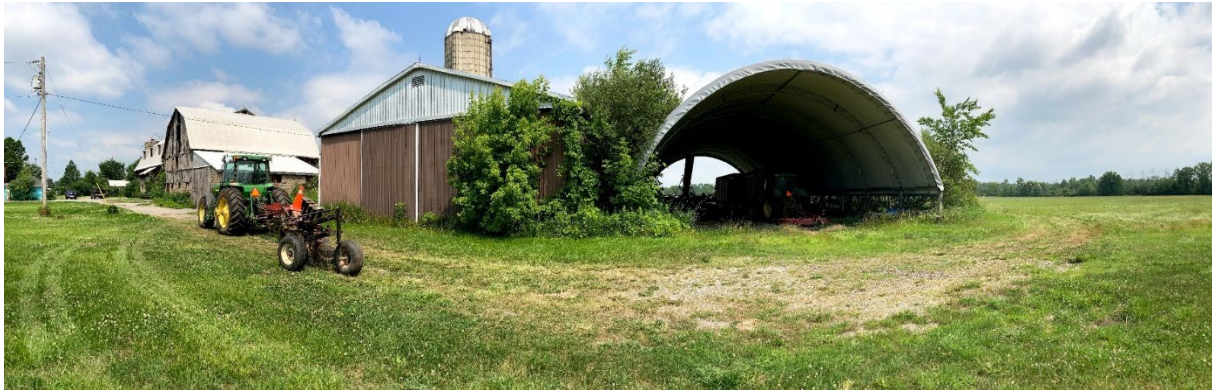
Plate 12: View of the circulation routes surrounding Outbuilding 3 and the Quonset, facing north
