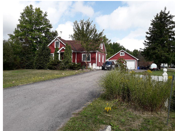
Plate 16: Northwest view of 7197 Reixinger Road
