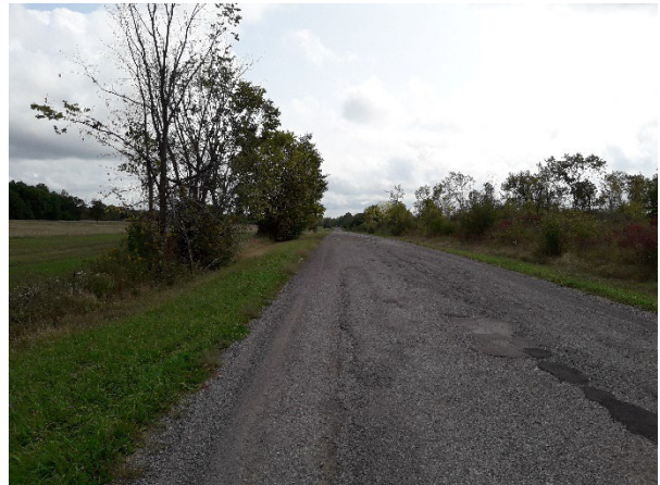
Plate 2: East view of Reixinger Road
