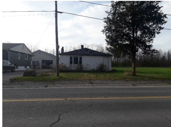
Plate 34: West view of 8825 Montrose Road (RR98)
