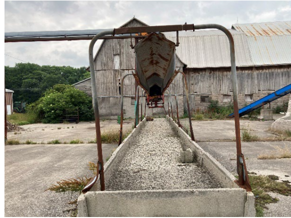
Plate 60: Metal conveyor attached to the north elevation of Barn 1
