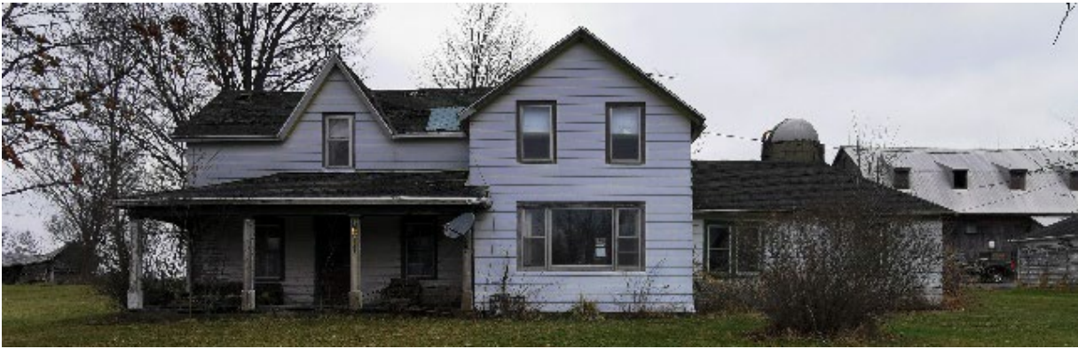
Plate 40: Front façade (south elevation) of 6811 Reixinger Road
