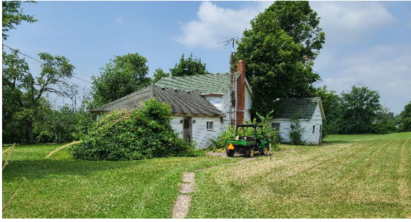
Plate 51: Photo showing north and east elevations of 6811 Reixinger Road
