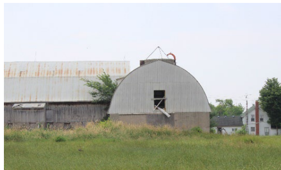
Plate 92: Barn 2 with concrete foundations/blocks and aluminium roofing, north elevation
