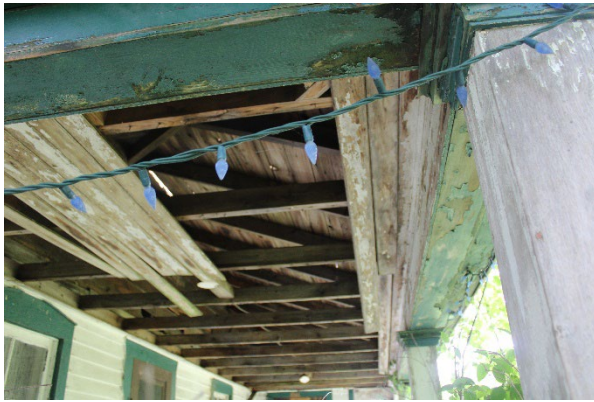
Plate 45: Underside of the covered veranda on the south elevation
