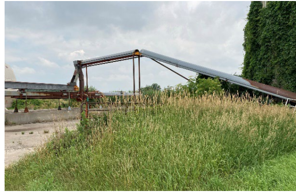
Plate 58: Metal conveyors located on the north side of Barn 1
