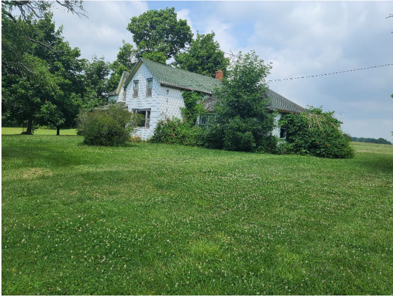
PHOTOGRAPH 3 View facing northwest towards 6811 Reixinger Road from rear field.
