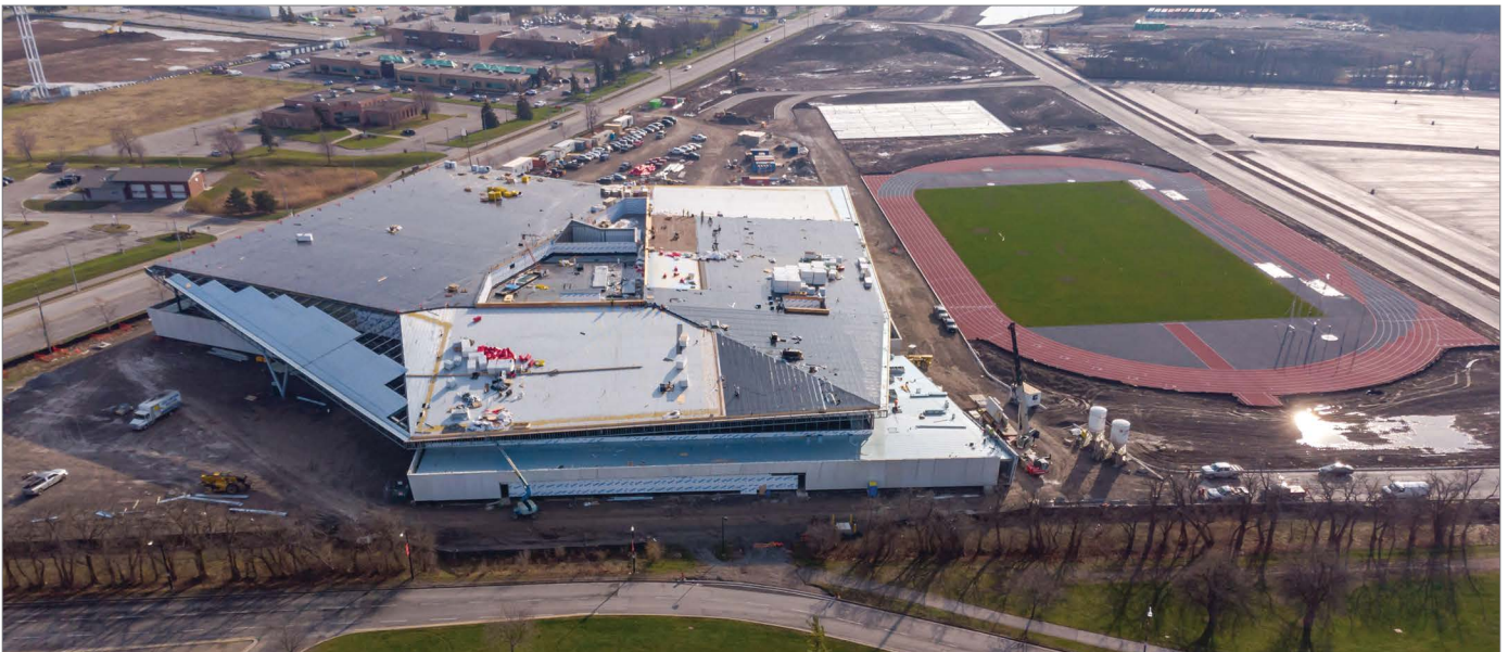
Canada Games Park under construction
